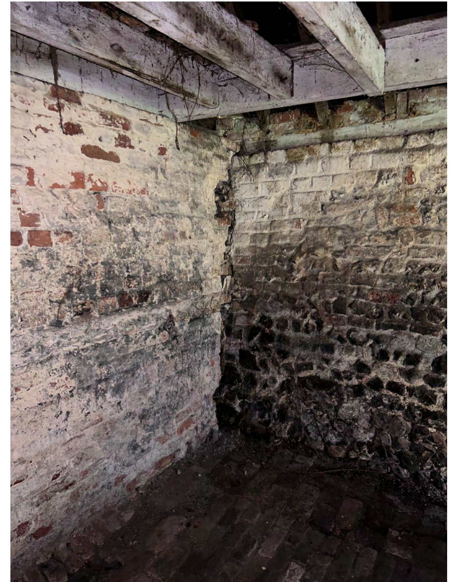
Fig. 14, Brick paviour floor and internal walls.
