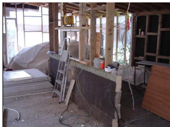
Figure 2 - 2009 construction photograph of 'Dayroom'
