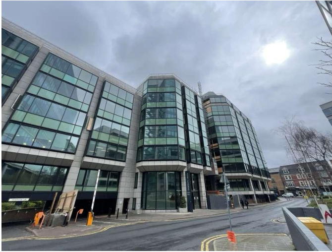
Photo 1: Western elevation of B1
