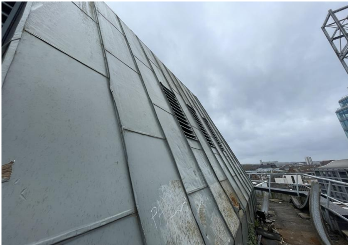
Photo 3: Roof of B1, to the north
