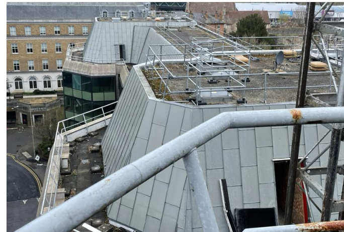
Roof of the plant room of B1
