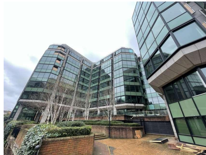
Eastern elevation of B1
