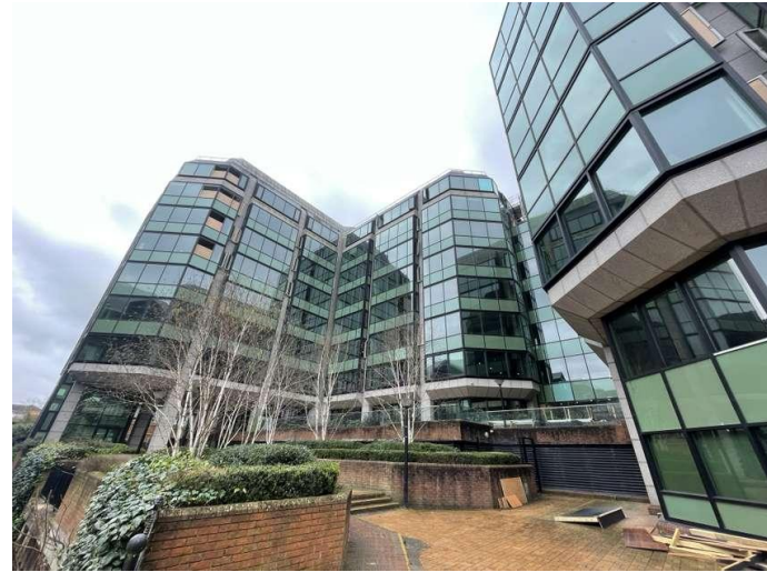
Photo 2: Eastern elevation of B1
