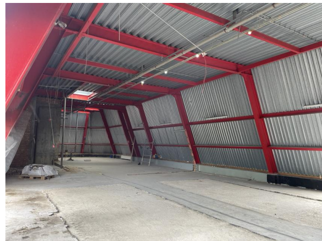
Photo 4: Internally within the roof of B1, to the south
