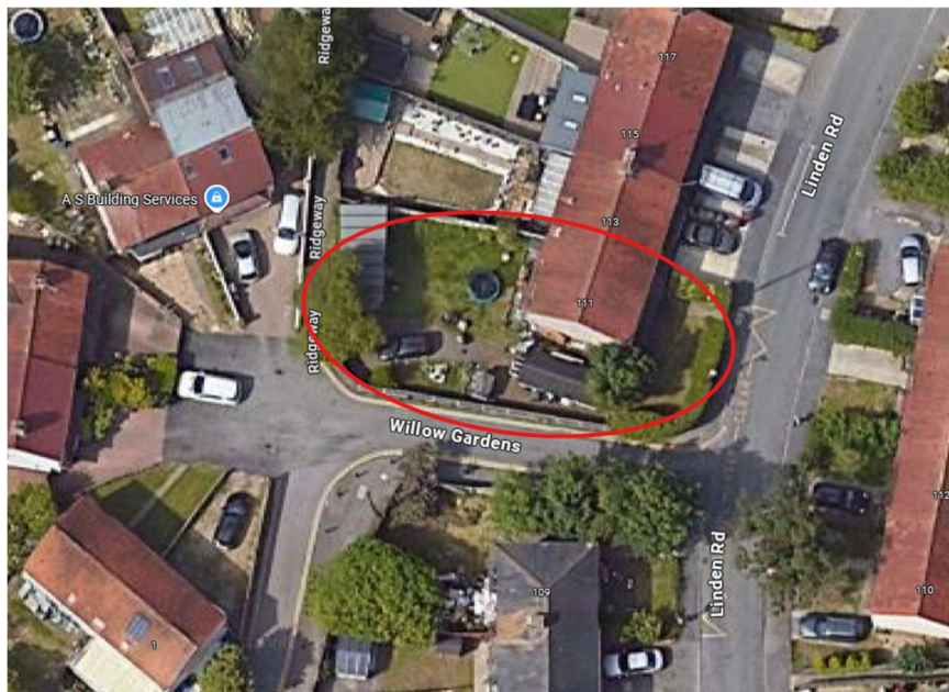
AERIAL IMAGE WITH SITE LAYOUT CIRCLED IN RED
