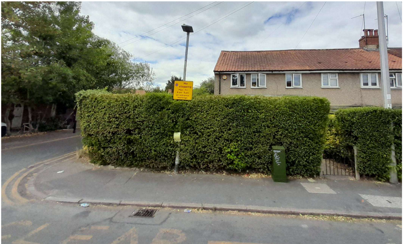
Looking west towards front elevation of host property
