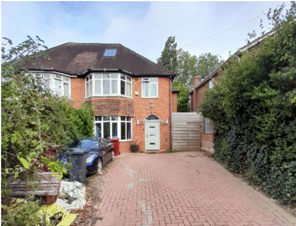
Looking towards south facing, front elevation
