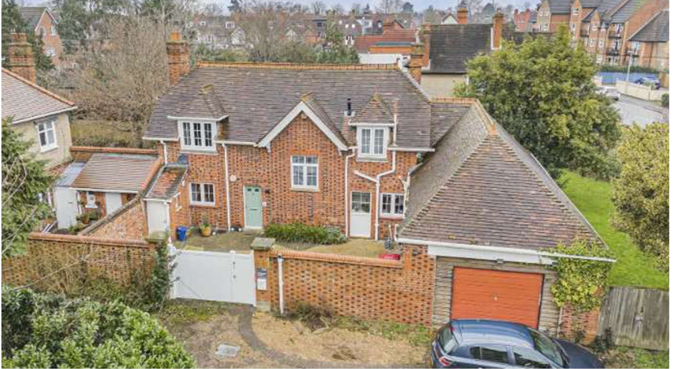
Looking towards front elevation set behind gates within courtyard.
