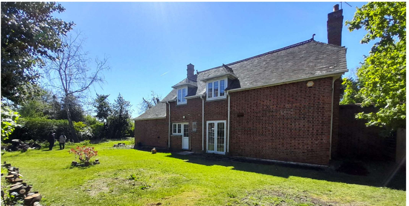
Rear elevation and rear garden
