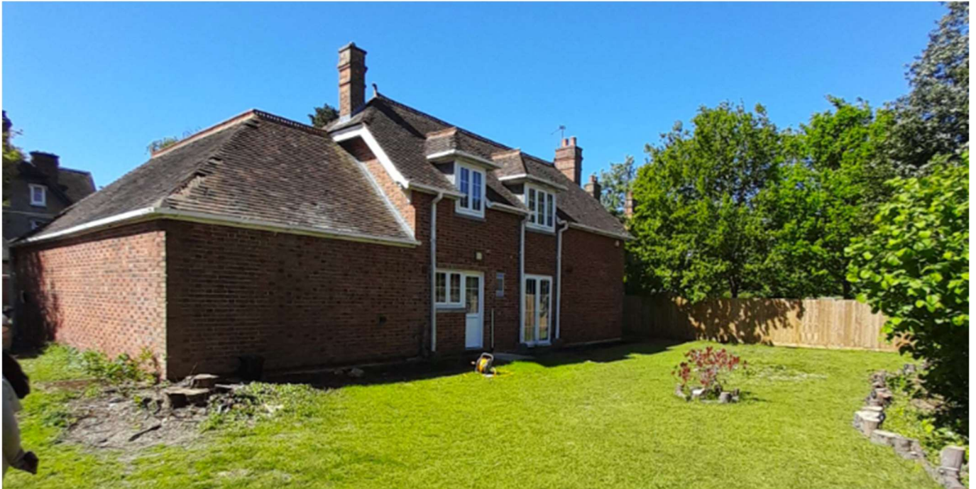
Looking towards north-easterly facing rear elevation
