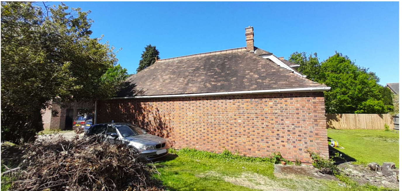
Looking towards existing garage and south-easterly facing elevation
