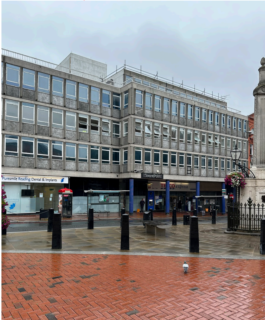
Photograph taken from Market Square - Section 1 on previous page Existing condition before the demolition works started. The new lift overrun will be substantially lower than the original lift enclosure.
