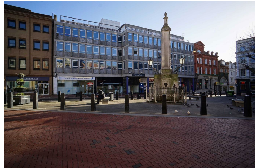
Figure 2 Front elevation facing the Market Place, 2021
