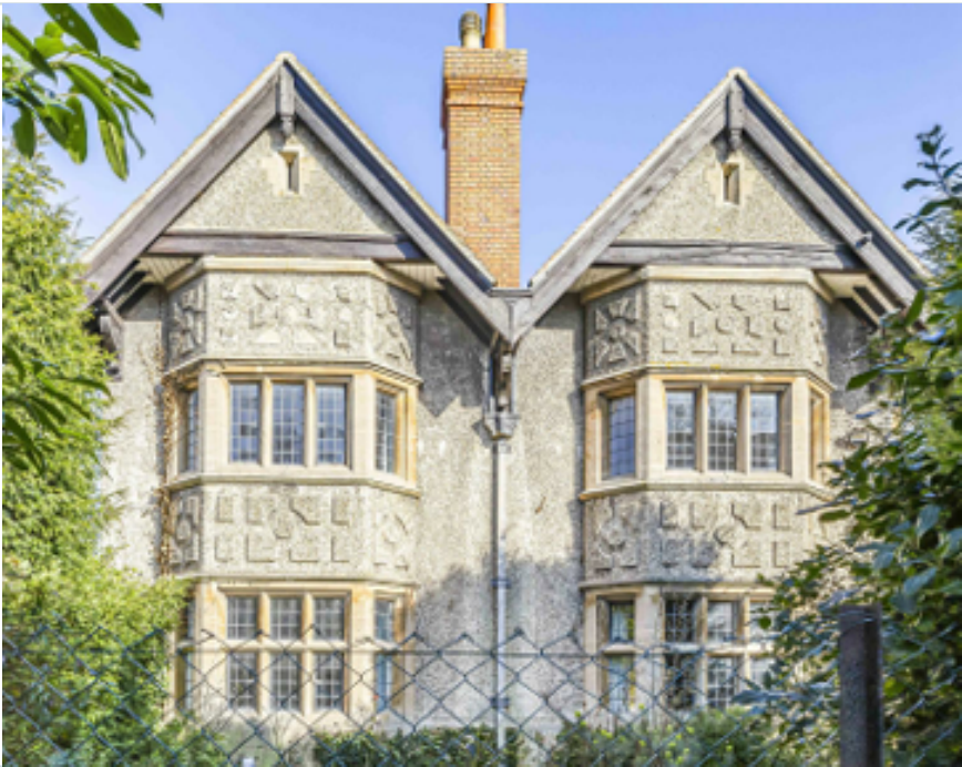
PHOTO: EXISTING FACETED 1 + 3 + 1 BAYS
