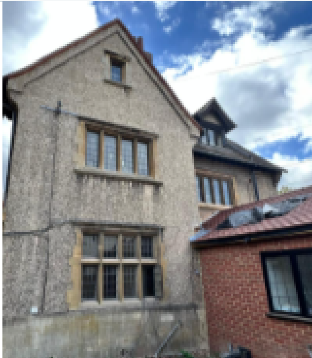
SIDE 1 / GABLE & GROUND
