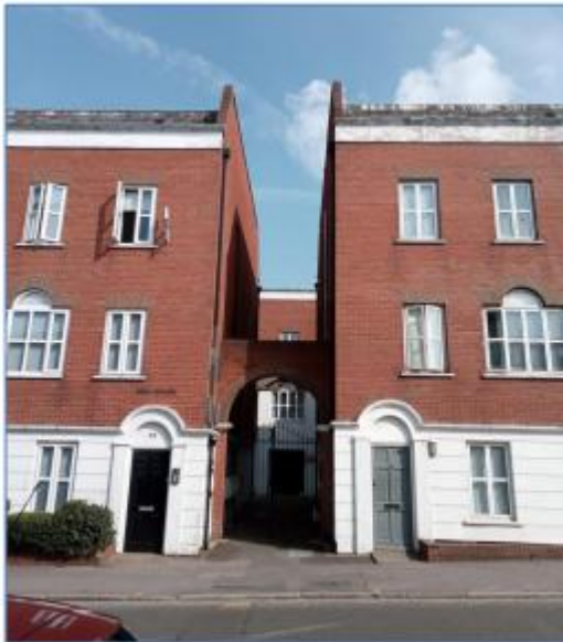
Site in street scene
