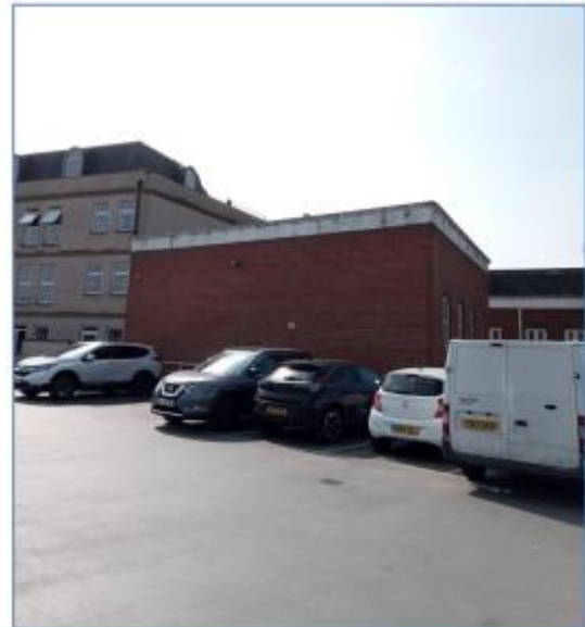
Rear of Site
