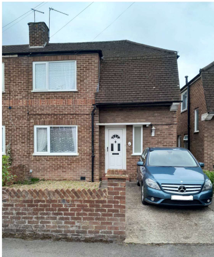
Looking towards the north facing – front elevation
