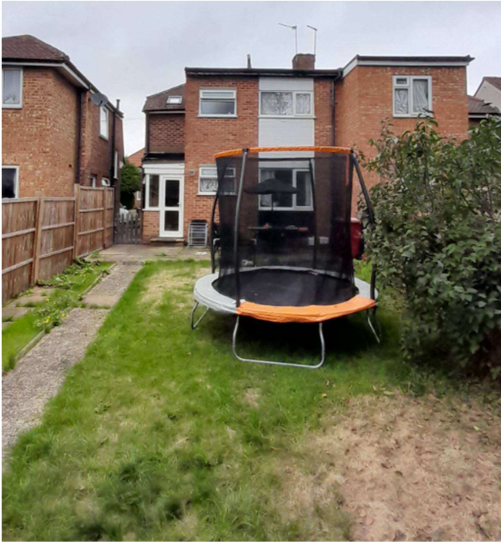
Looking towards the south facing – rear elevation
