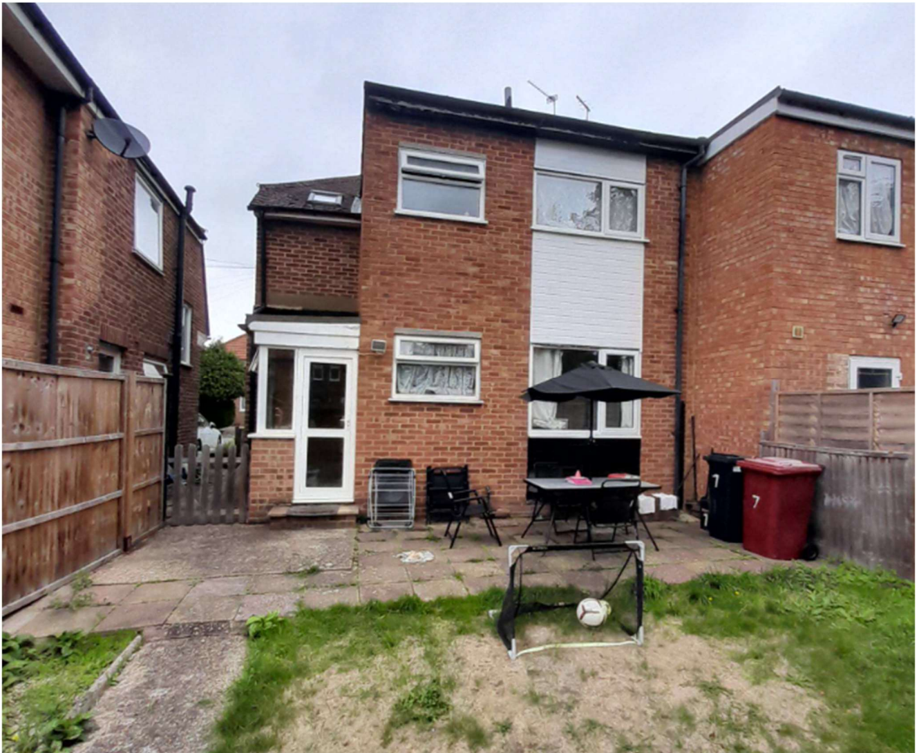
Looking towards the south facing – rear elevation
