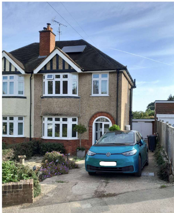
Looking towards south-westerly facing – front elevation.
