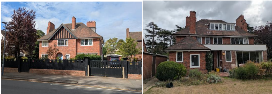
Left: Site frontage, photo taken by case officer on 19 August 2026.
