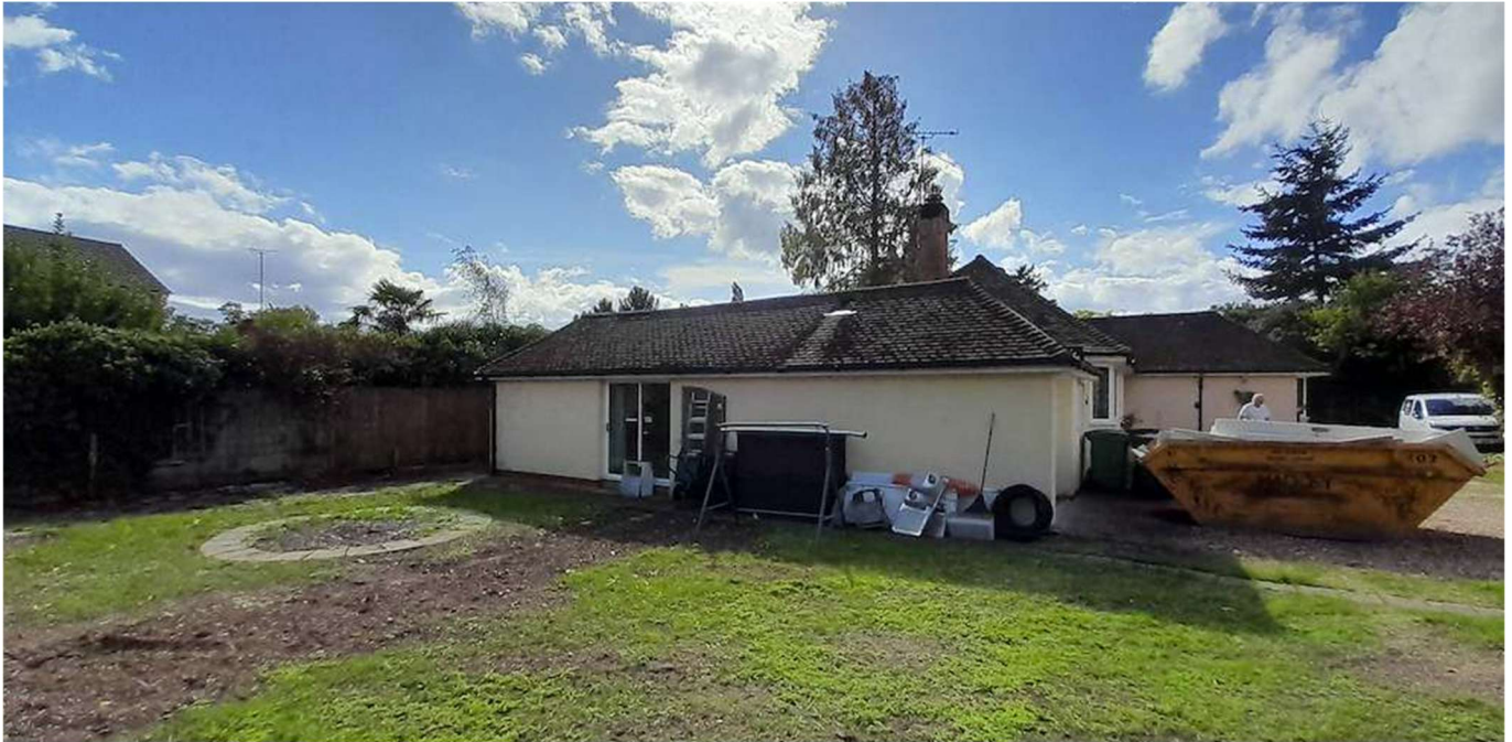
Looking towards existing north facing side elevation
