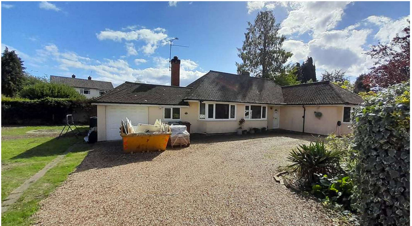
Looking towards the existing west facing front elevation
