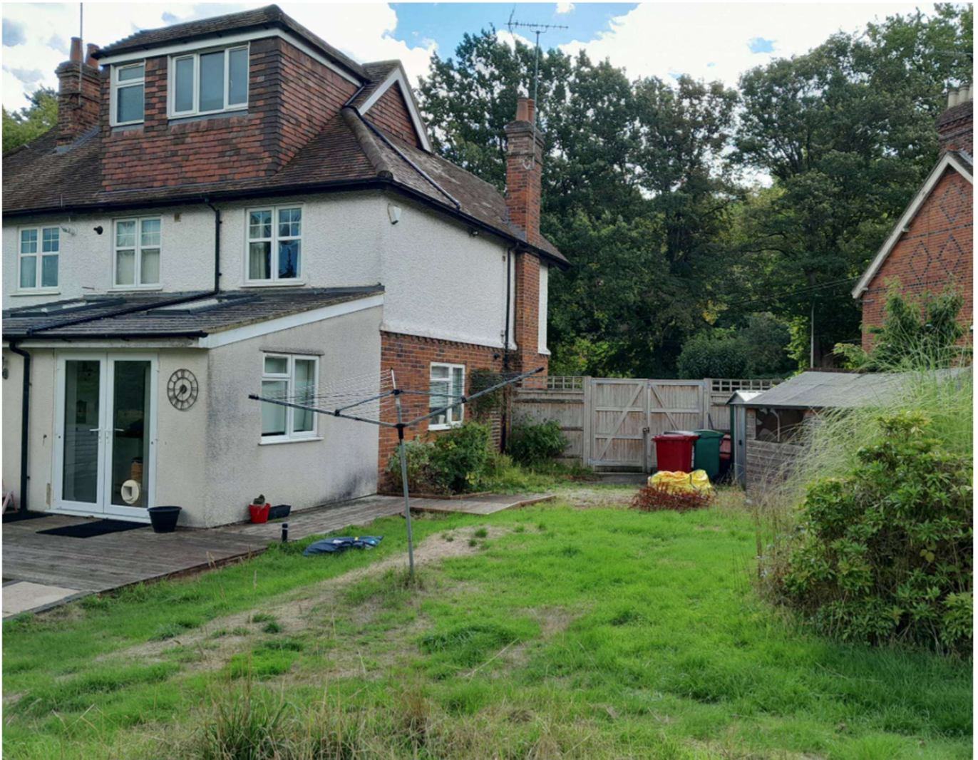
Looking southeast towards the rear / side elevations of the host property
