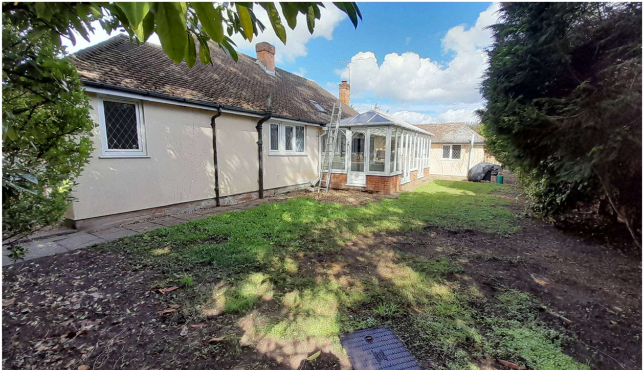
Looking towards existing conservatory (to be demolished) and rear elevation
