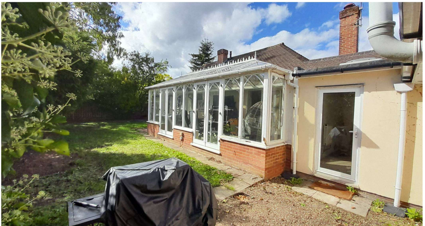
Looking towards existing conservatory (to be demolished) and rear elevation
