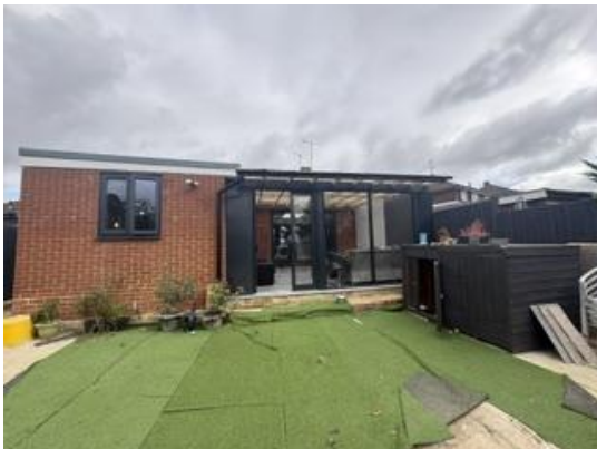
Looking towards the outbuilding and the linked rear extension
