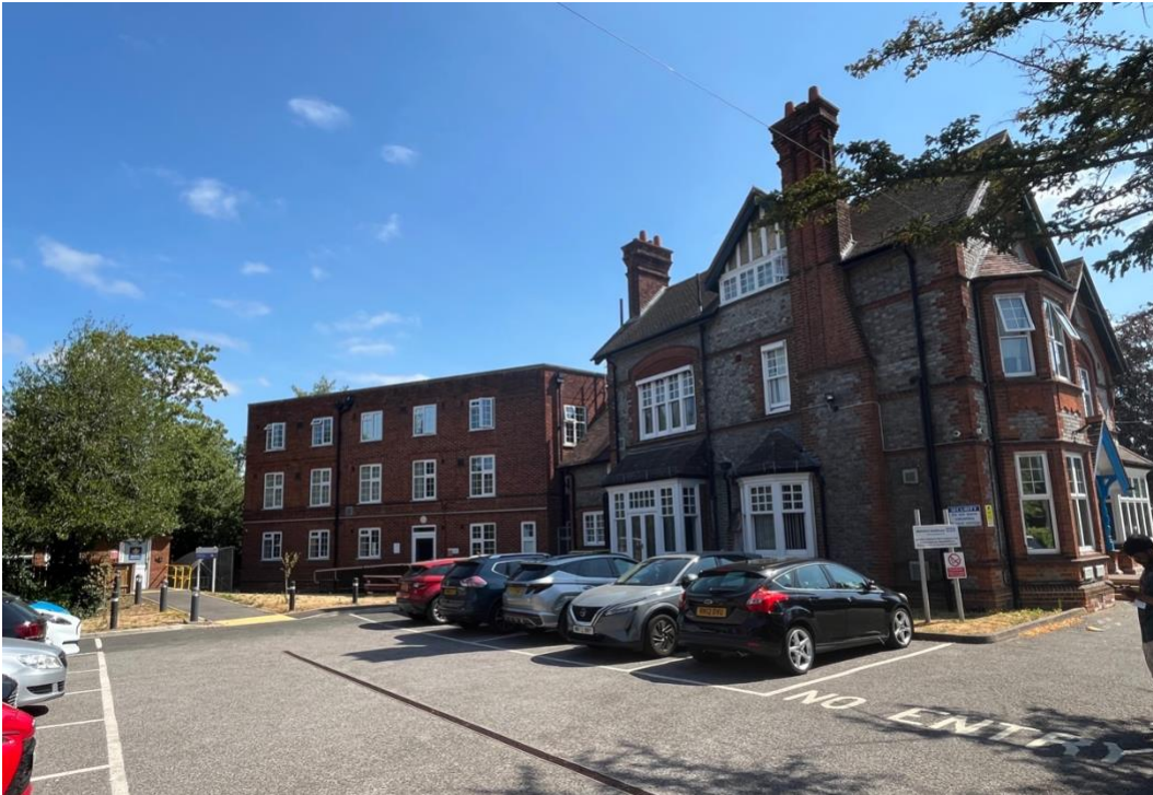
Figure 6: The two blocks at 25 Erleigh Road – the older 19 th -century house at the front of the site and the 1939 block as a rear extension to this older structure
