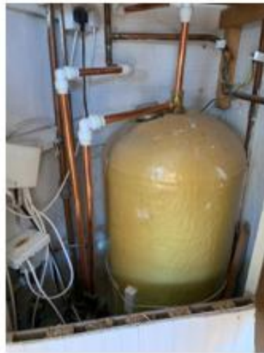
Fig 7a Internal pipework (historic north east wall, bathroom side)
