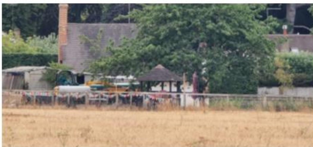
Fig. 8 View from the public right of way to the northwest of the listed building, showing the extant garage and attached lean-to structures and cherry tree partly obscuring and filtering views of the timber framing. OS PMCL AC0000855630
