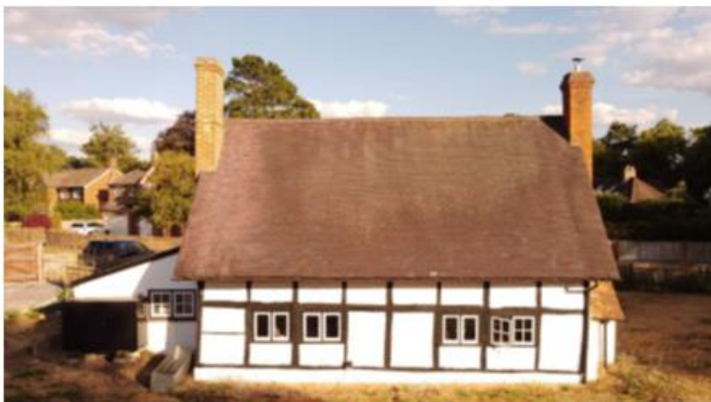
Fig. 6 Drone view showing the northwest elevation without the clutter of buildings and vegetation in the foreground. OS PMCL AC0000855630
