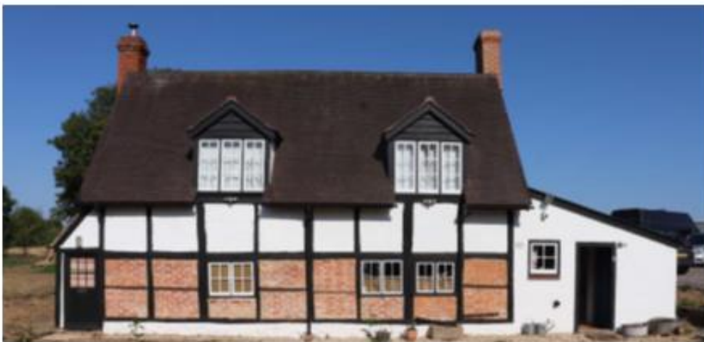
Fig. 3 The key southeast facing elevation of 3, Blagrove Lane, viewed from the lane. OS PMCL AC0000855630
