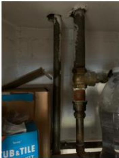
Fig 6a Internal pipework (historic north east wall, bathroom side).
