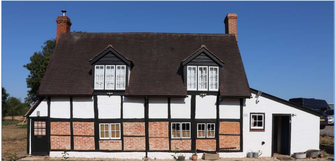
Fig. 12 The key southeast facing elevation of 3, Blagrove Lane, viewed from the lane. OS PMCL AC0000855630
