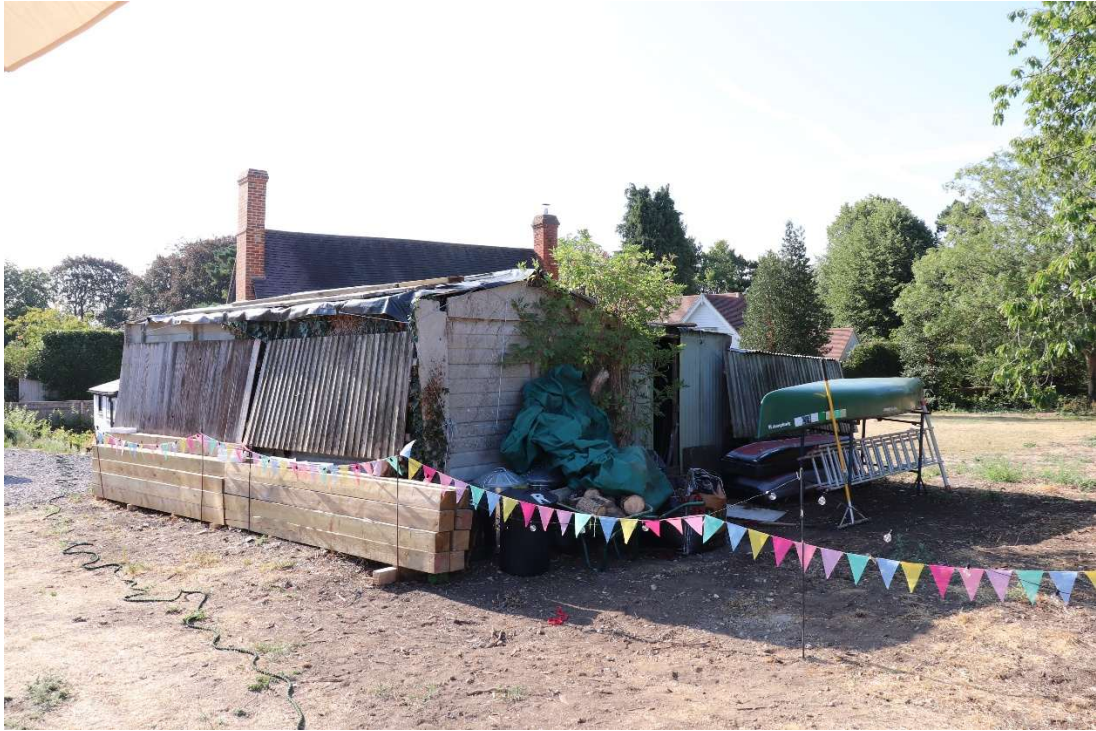
Fig. 17 Internal view from the northwest of the listed building, showing the extant garage and attached lean-to structures. OS PMCL AC0000855630
