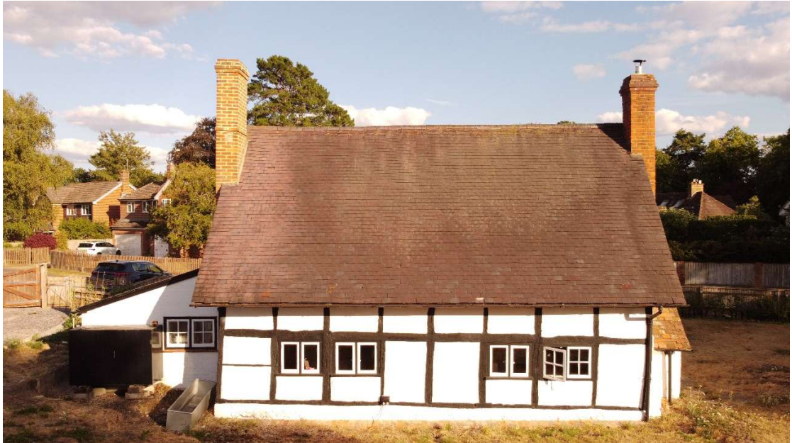
Fig. 15 Drone view showing the northwest elevation without the clutter of buildings and vegetation in the foreground. OS PMCL AC0000855630
