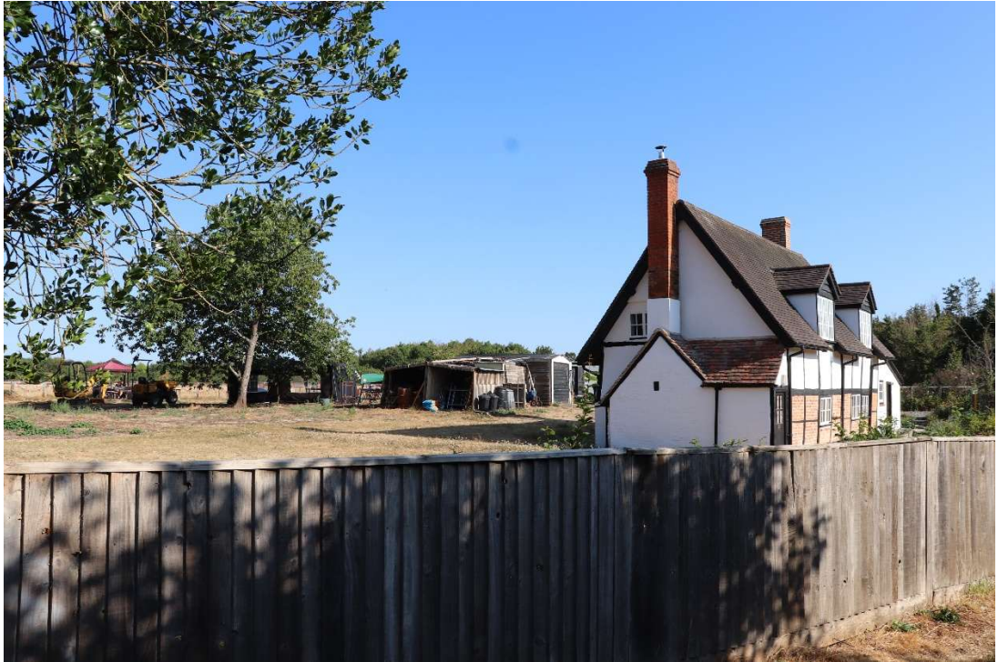
Fig. 14 View looking along Blagrove Lane from the south, with existing garage and attached lean-to structures seen to the left of the cottage. OS PMCL AC0000855630
