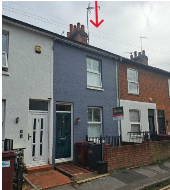
Photo 1 – View of front elevation (west)
