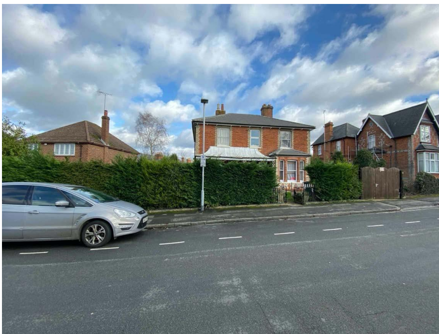
Street view, showing the site in its wider context
