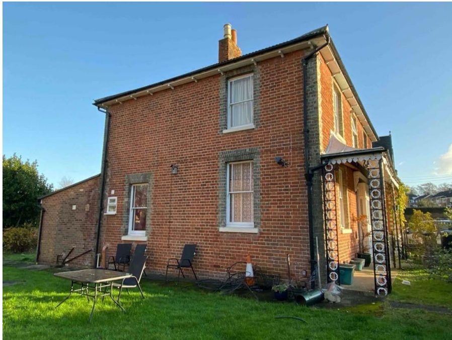
Side and rear elevations – the extent of the later single storey additions
