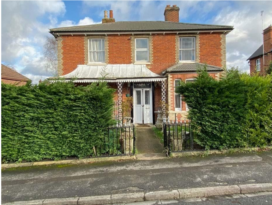
Front elevation from Hamilton Road – to be retained unaltered
