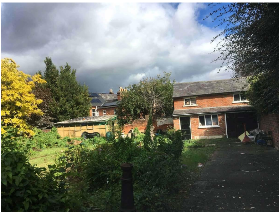
Outbuilding and adjoining storage shed
