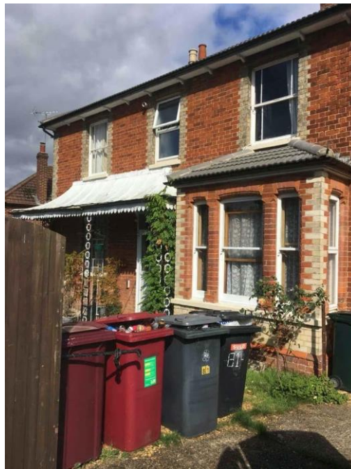
Front elevation – surviving verandah and later bay
