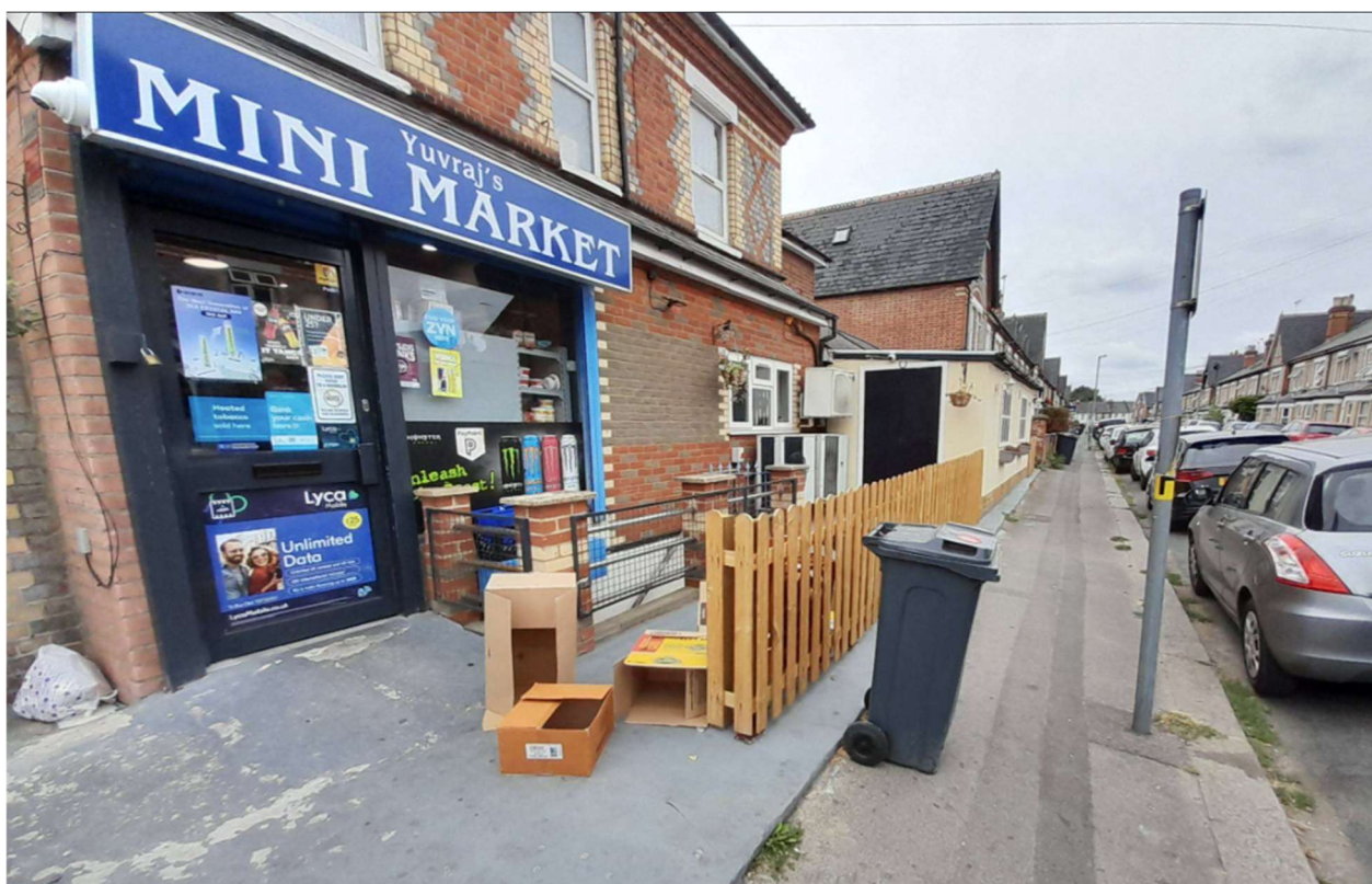
Looking southwest towards side elevation with unauthorised structure in background.
