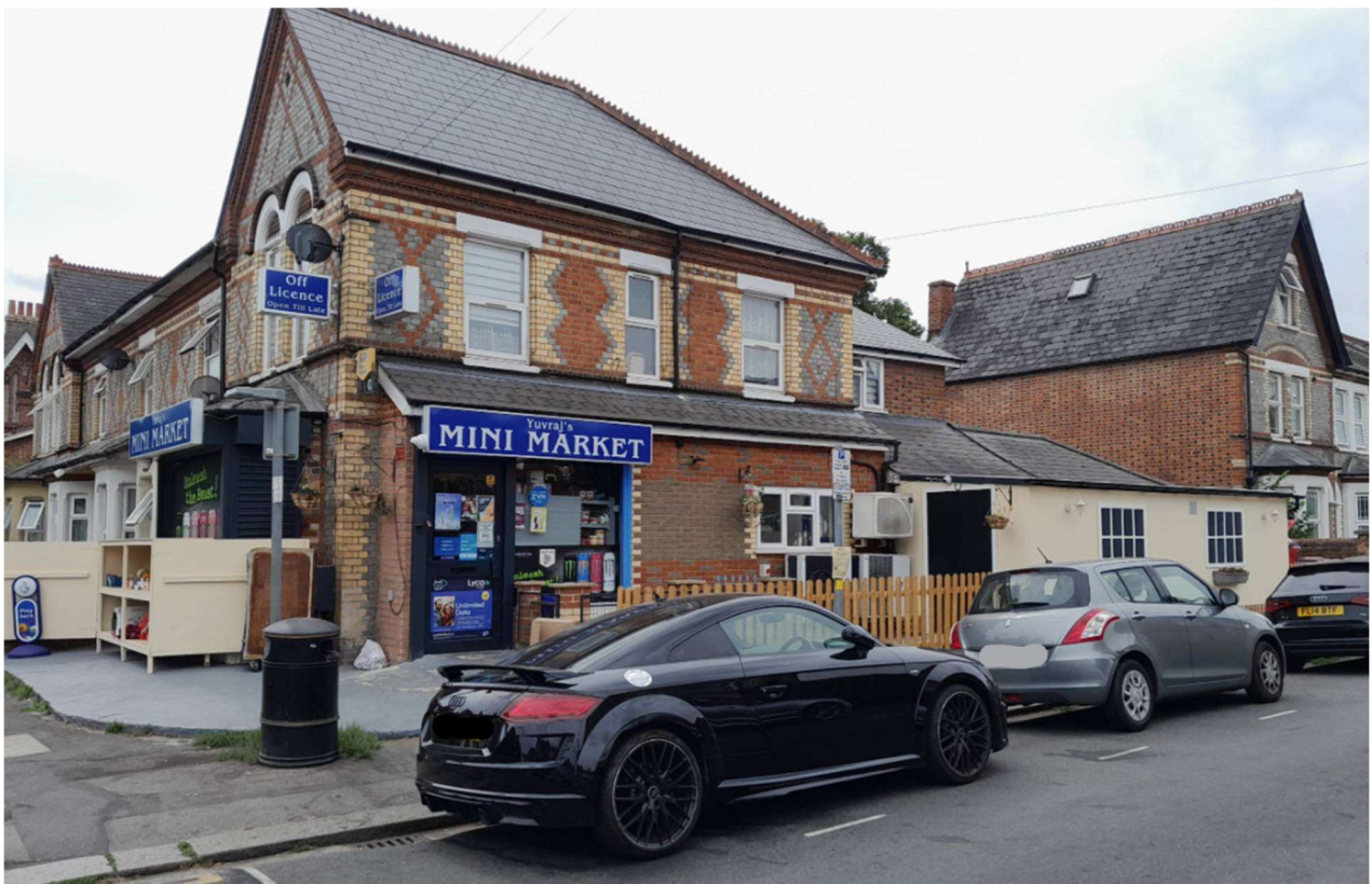
Looking south towards side elevation facing Radstock Road
