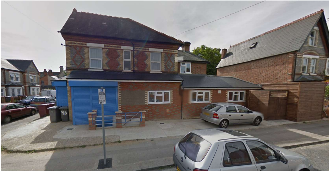
Radstock Road (side) elevation with unauthorised timber structure on the right-hand side of image, dated 2012
