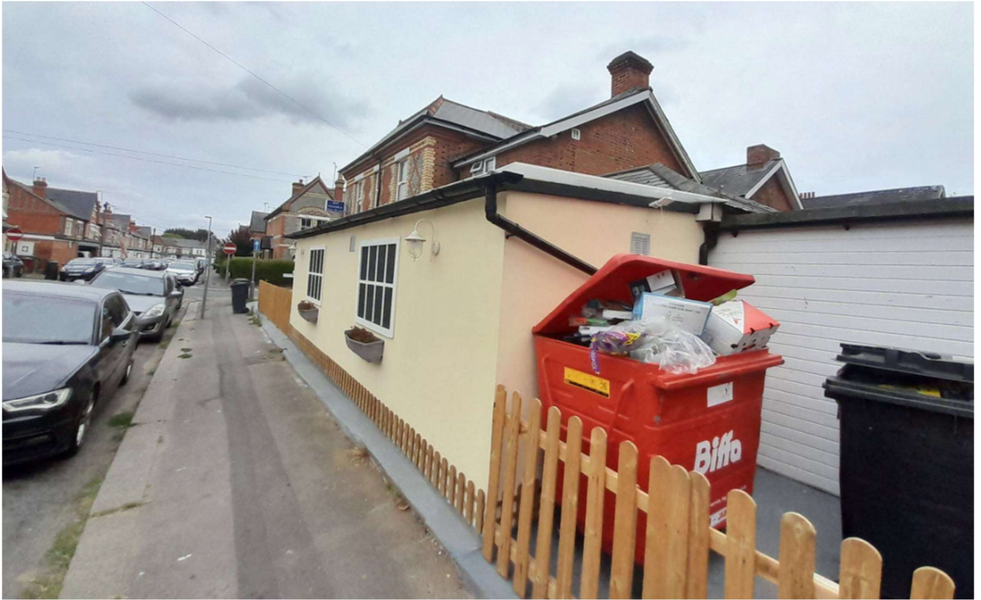
Looking northeast towards unauthorised structure facing Radstock Road.
