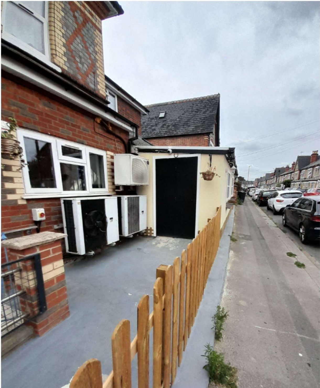
Looking southwest towards unauthorised structure.
