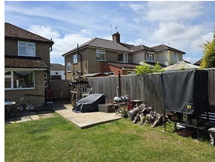
Existing view to No. 50
