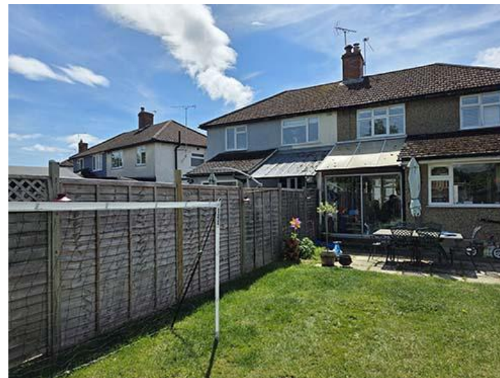
Existing view to No. 46
