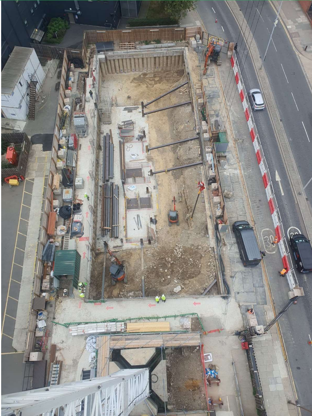
Example of Pit lane details with secure mesh gates and fencing on all sides. Traffic Marshal shown in Orange PPE
