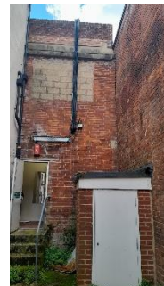
View from ground floor of surrounding walls to the enclave space
