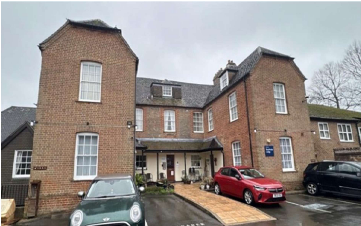
Looking towards the front (main entrance) elevation.
