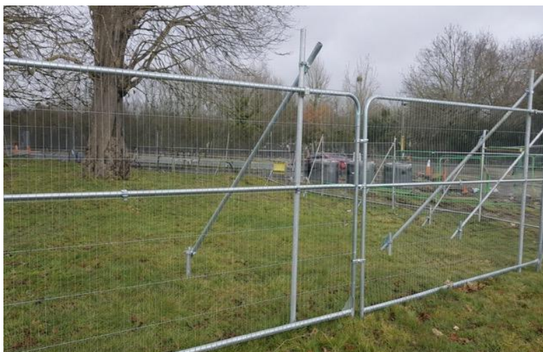
TPB 1 — Scaffold framework with weld mesh panels and back-stays
