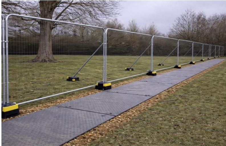
Ground protection example — wood chip and trackmats
