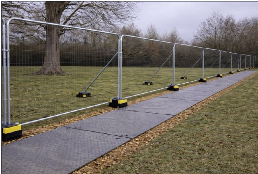
Ground protection example — woodchip and trackmats
