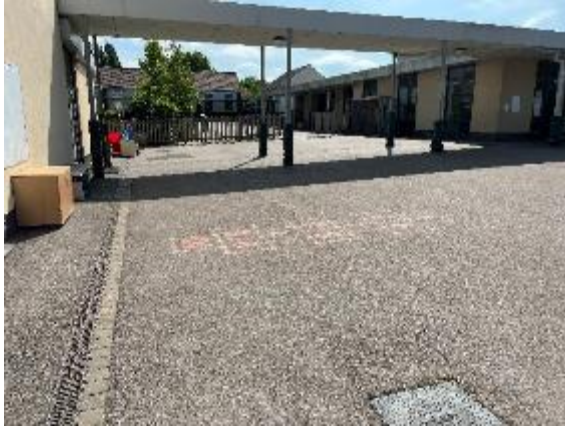
Photograph 3. Hard standing within the courtyard between the school buildings (u1b).
