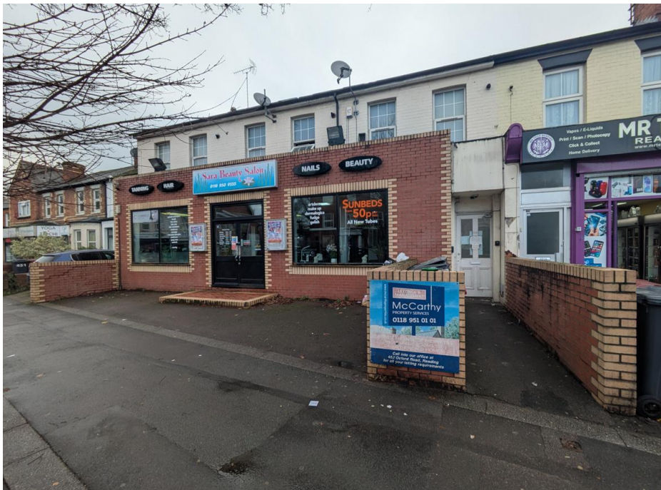
Figure 1 Photo of the front of the site taken from Oxford Road by the case officer on 19 November 2025
