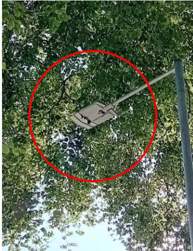
Indicative pruning to provide 1m clearance from lamp head
