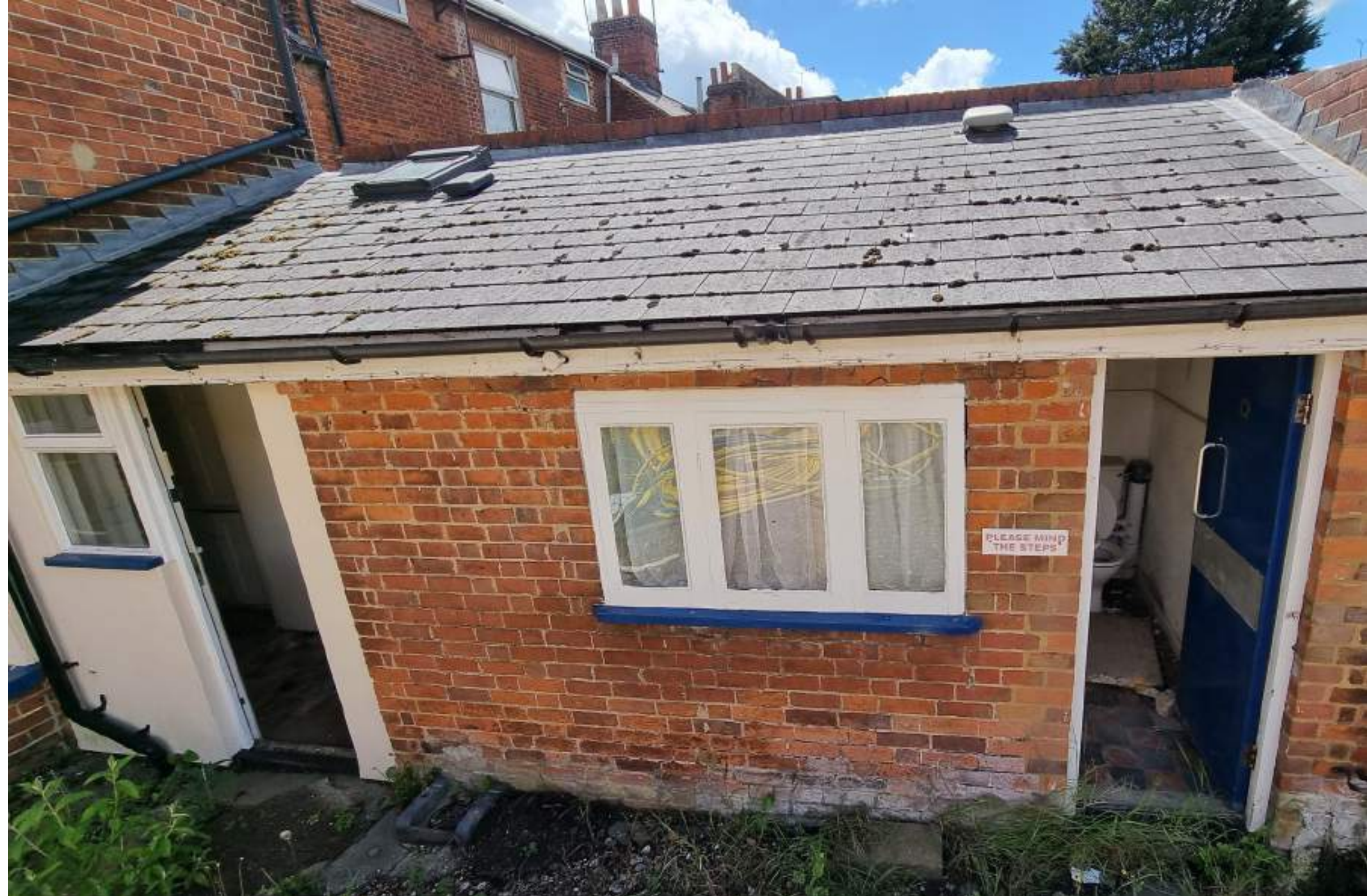
Remaining extension to the south. Half brick skin cannot be upgraded, and modern doors and windows and recent roof with rooflight
