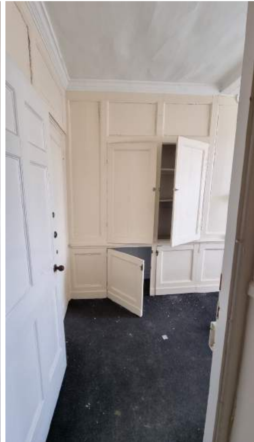
Small section of storage cabinets to be removed to install approved en-suite.
