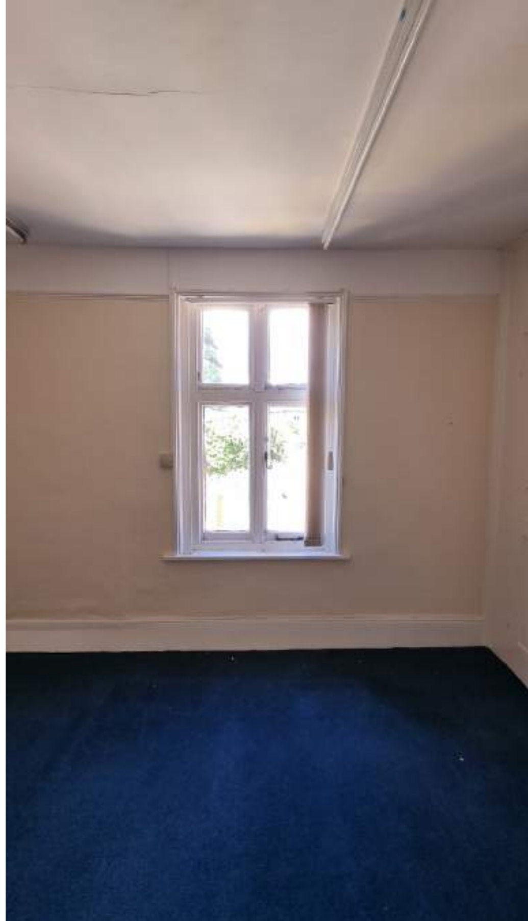
Existing ceiling and window
