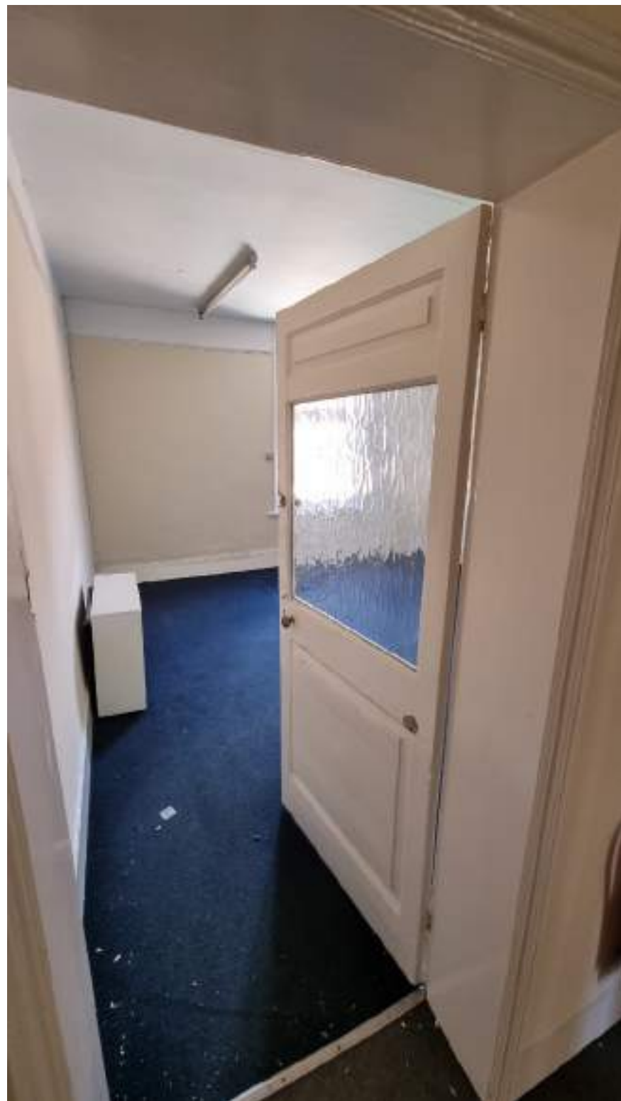
Door opening infilled as per approved application
