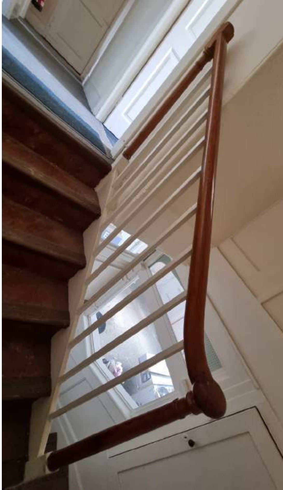
Handrails to be preserved.
