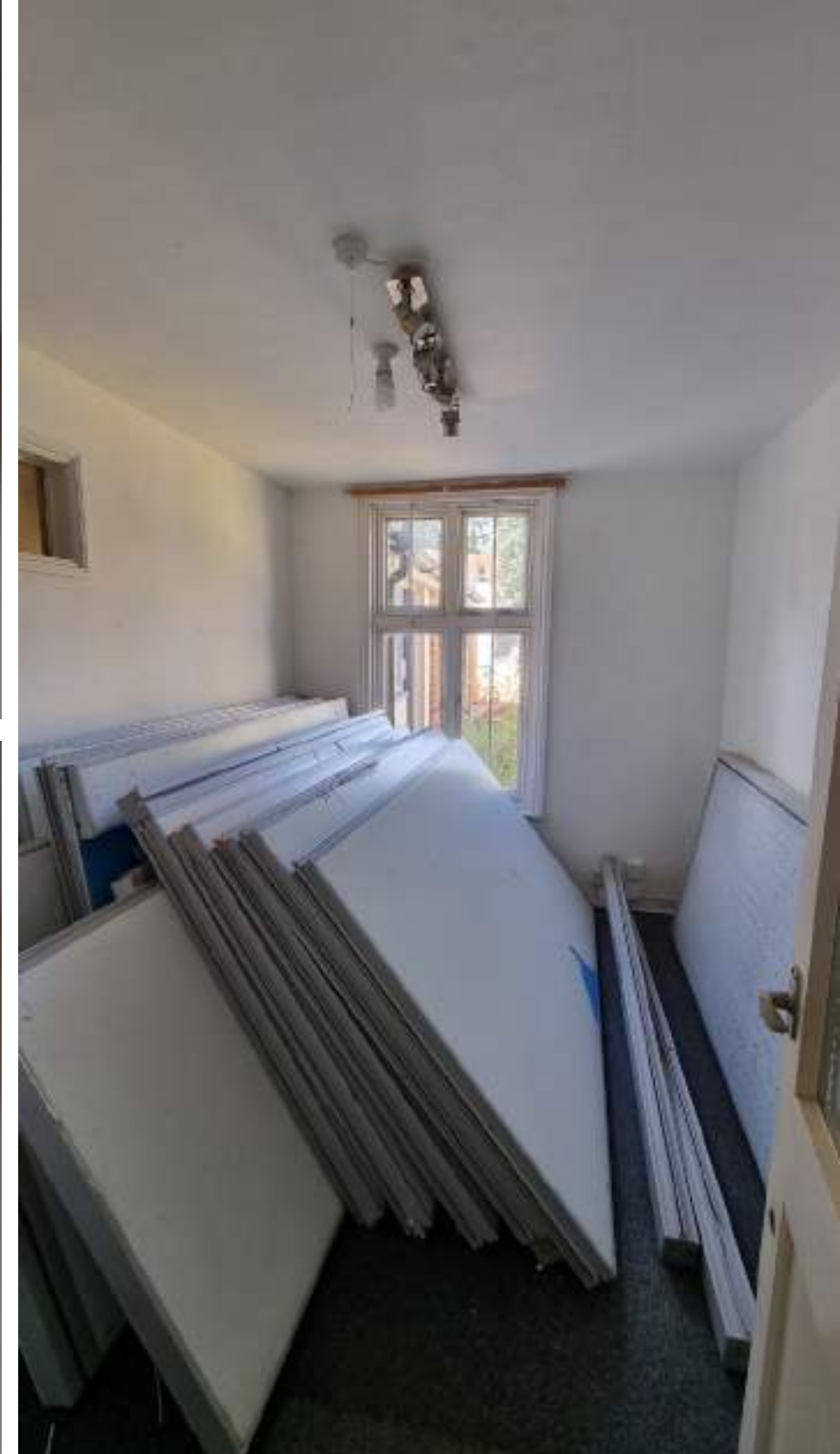
Existing plain walls, ceiling and floor, finishes appear to be modern. Window proposed to be retained.
