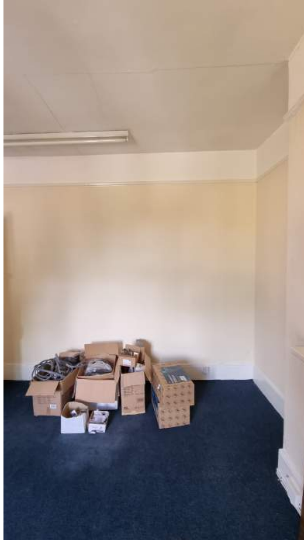
Wall between flat 4 and corridor - minimal detail
