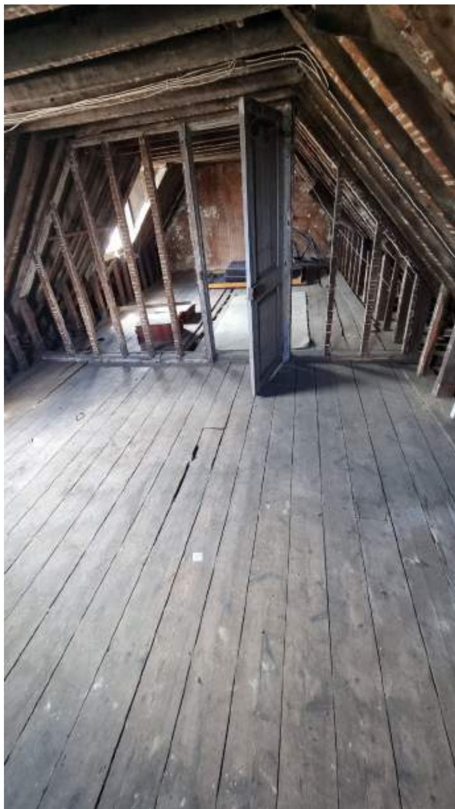
Unheated loft used as storage
