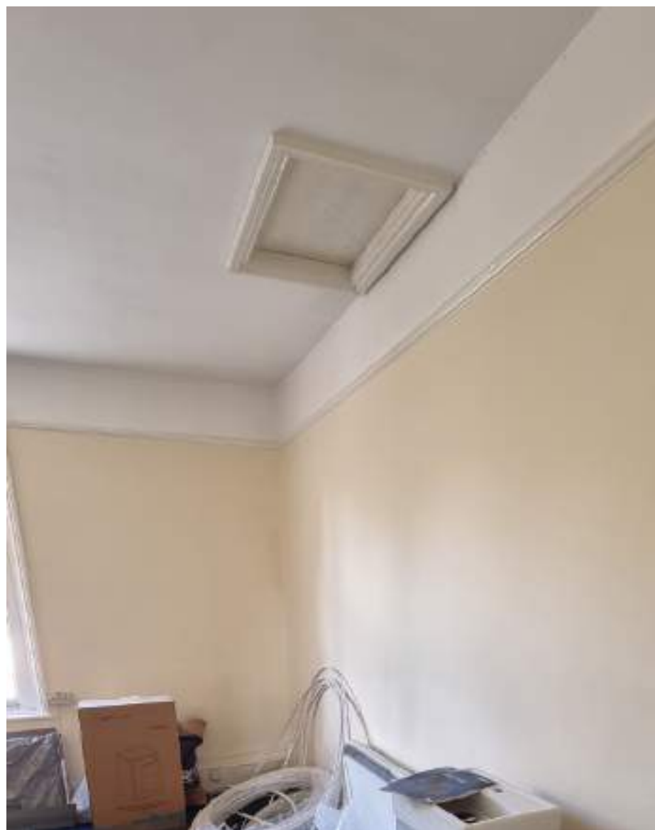
Existing ceiling, walls and loft hatch.
