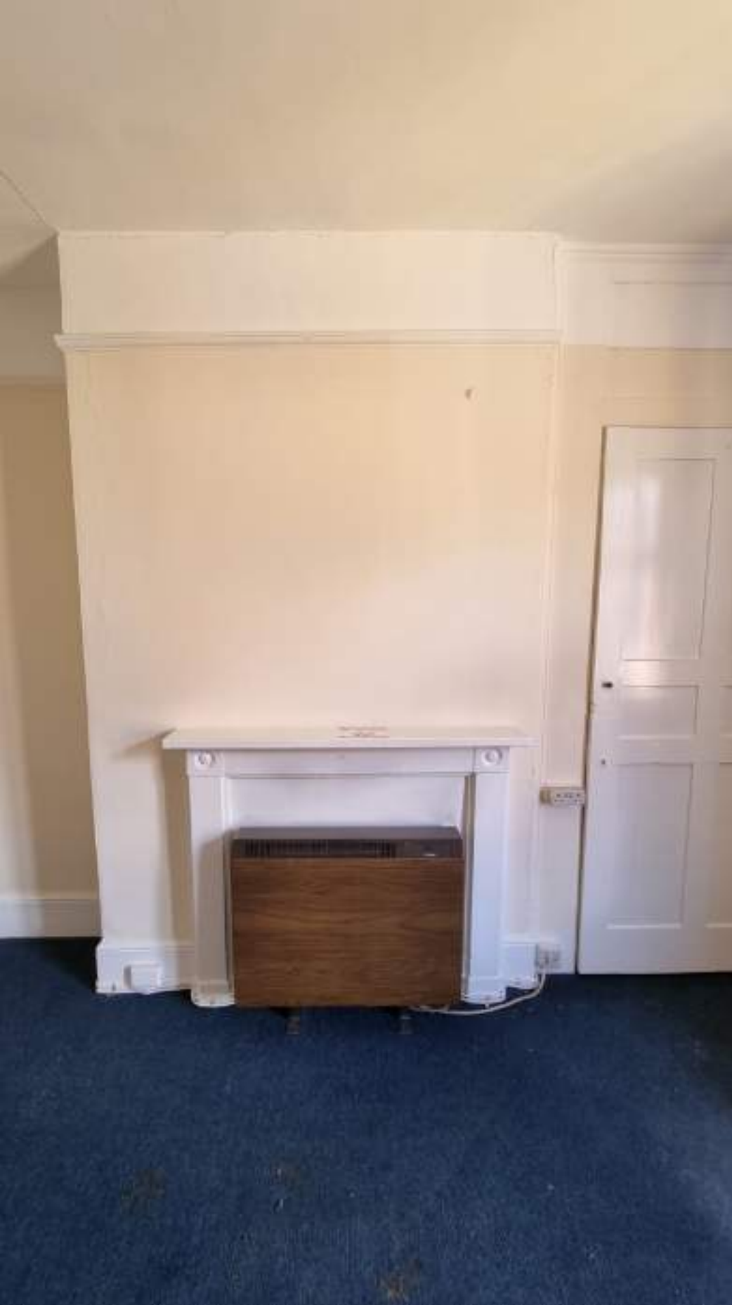
Chimney breast retained, modern heater removed
