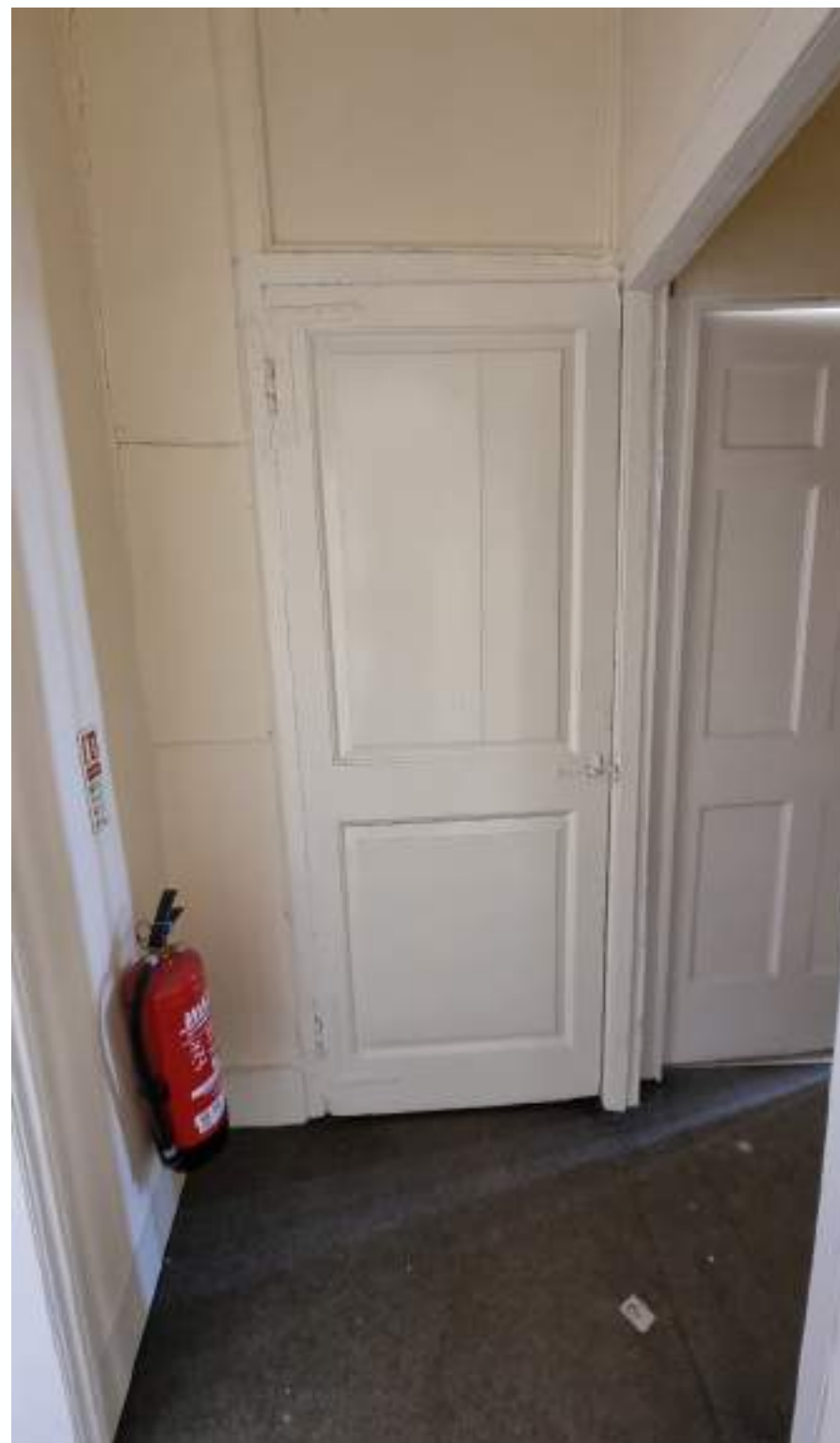
Door to loft storage
