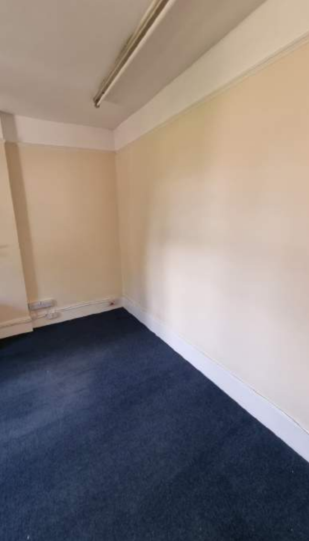
Existing walls to corridor
