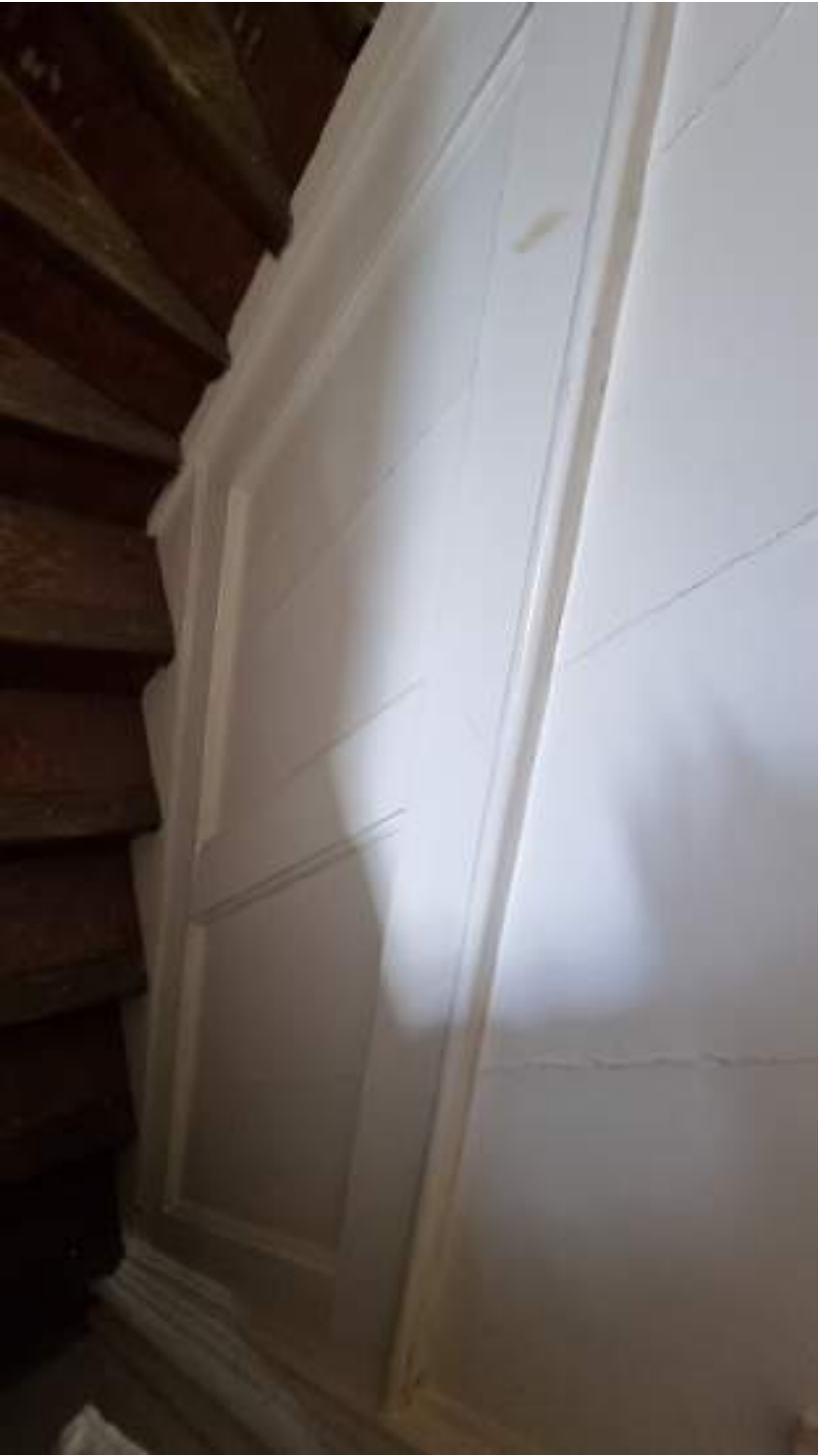
Timber panelling to the right
