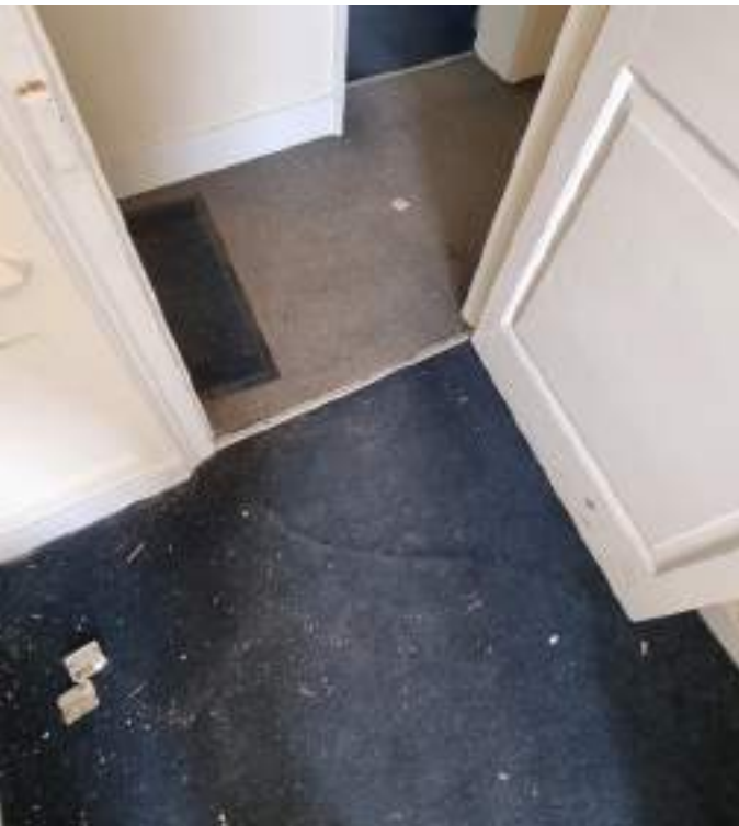
Existing carpet flooring replaced with carpet flooring.
