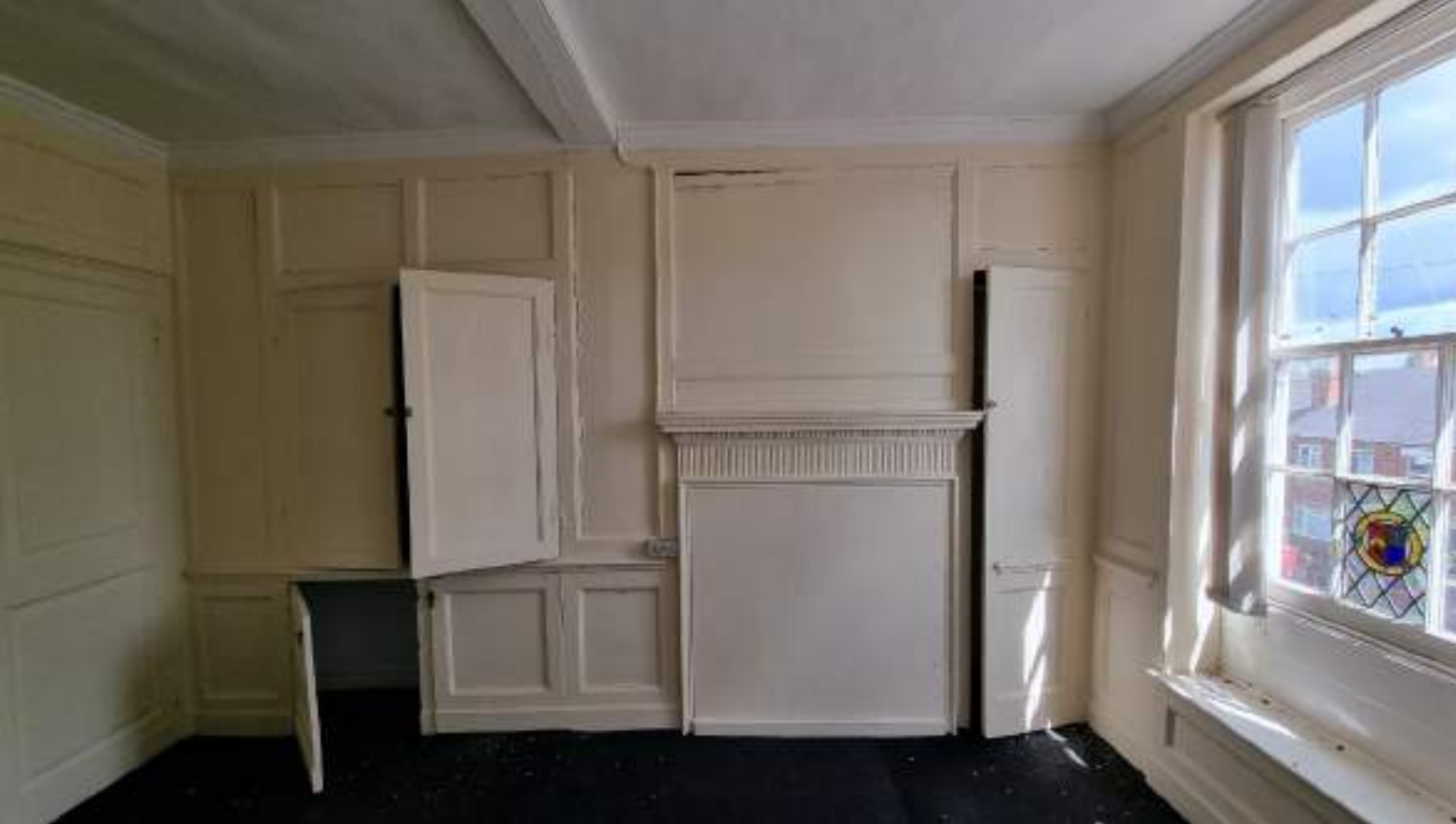
Full view of the panelling to north wall.
