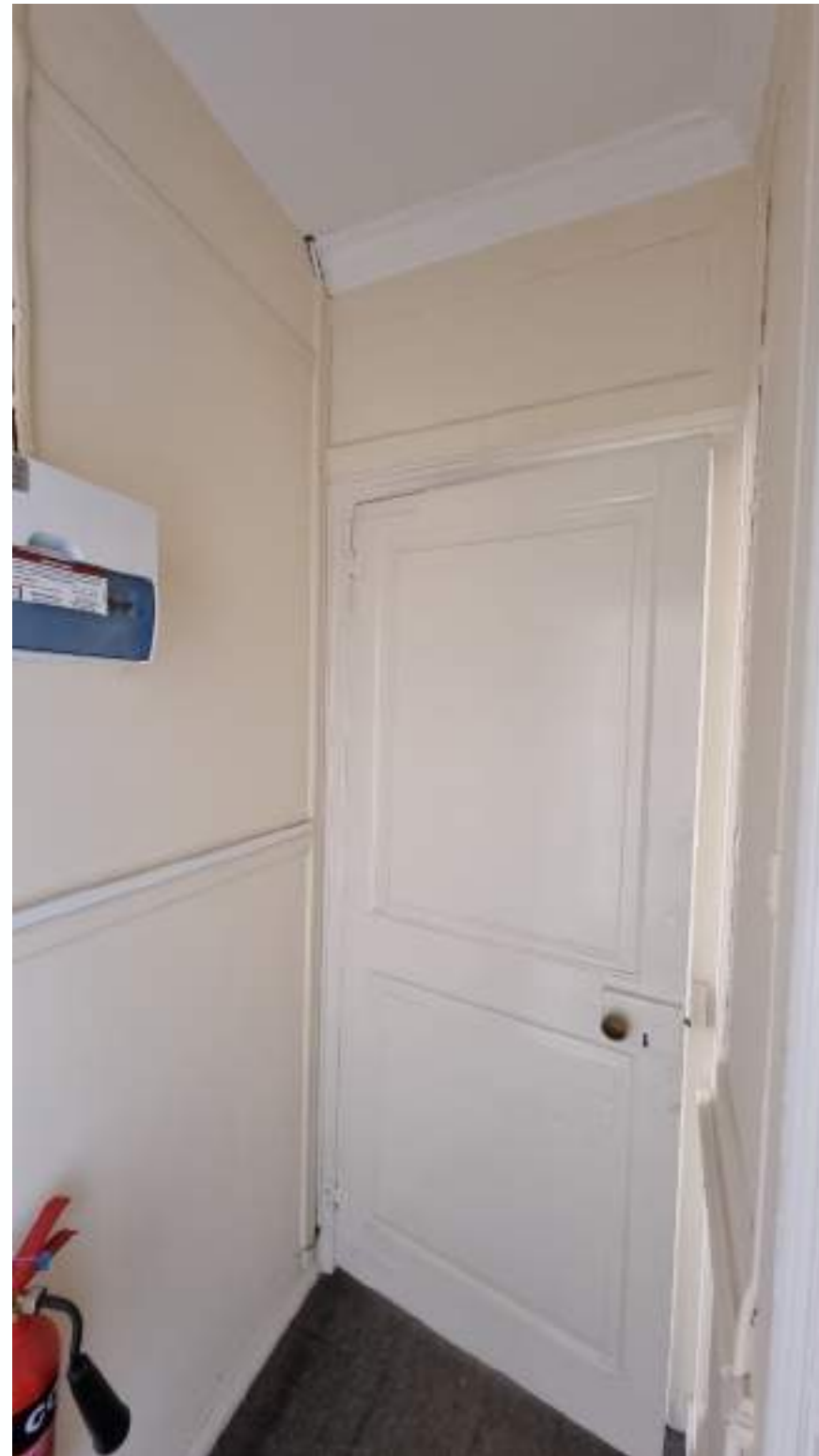
Existing door retained
