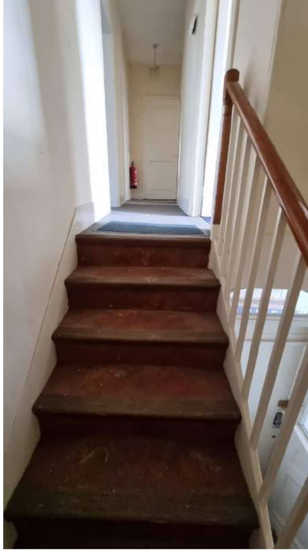
Modern corridor to first floor.
