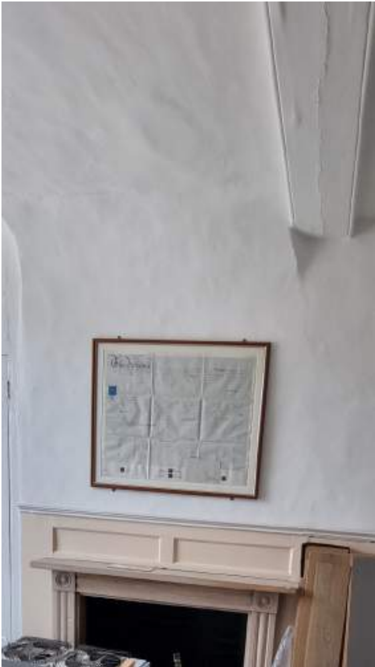
Existing chimney breast to be preserved, including timber panelling. Plain lath and plaster ceiling and timber beam above.
