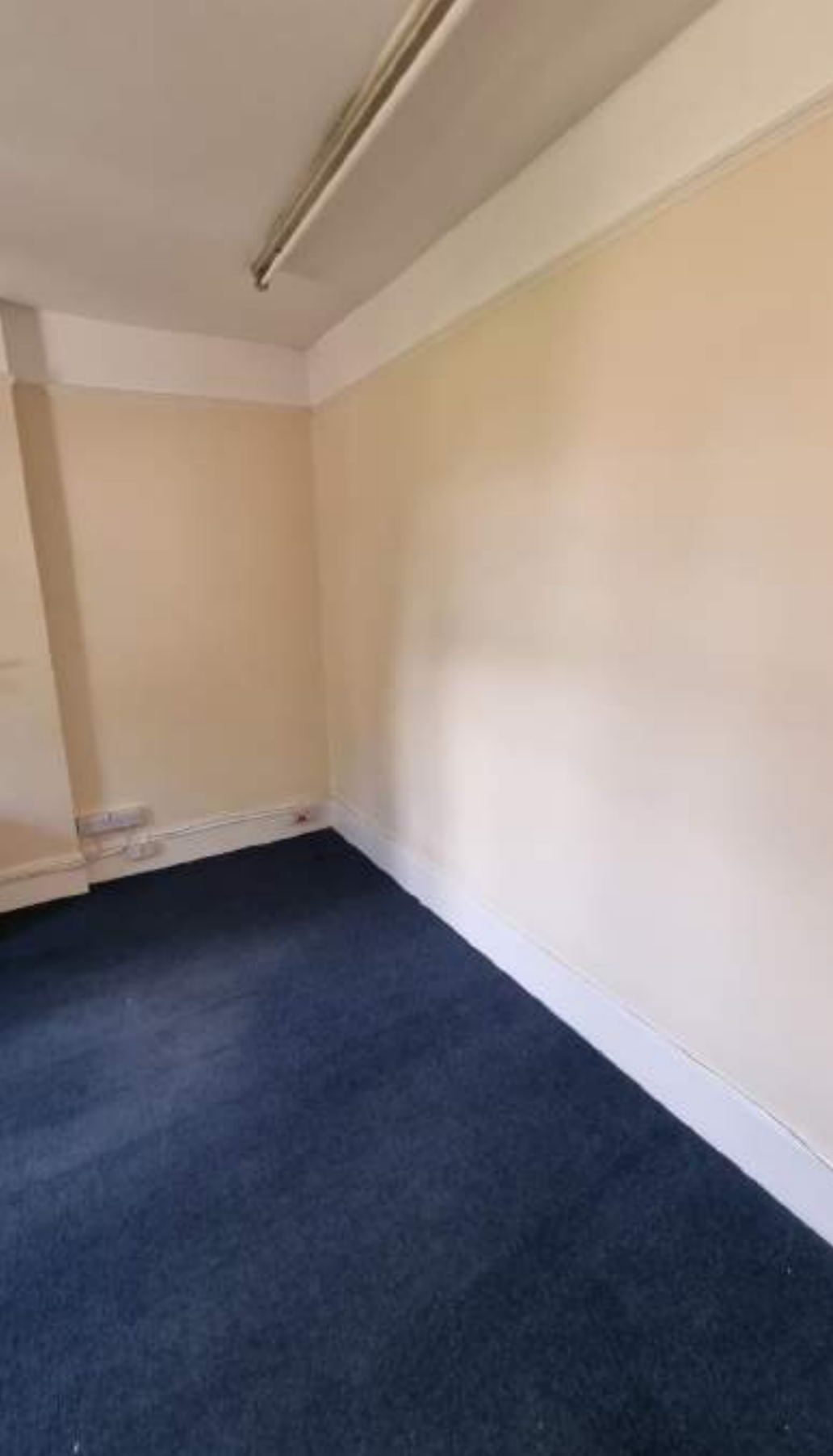
Existing walls to corridor
