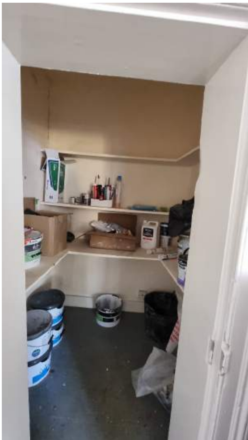
Inside the store. Shelving proposed to be removed. New access corridor to bedroom and wet room as per approved application.
