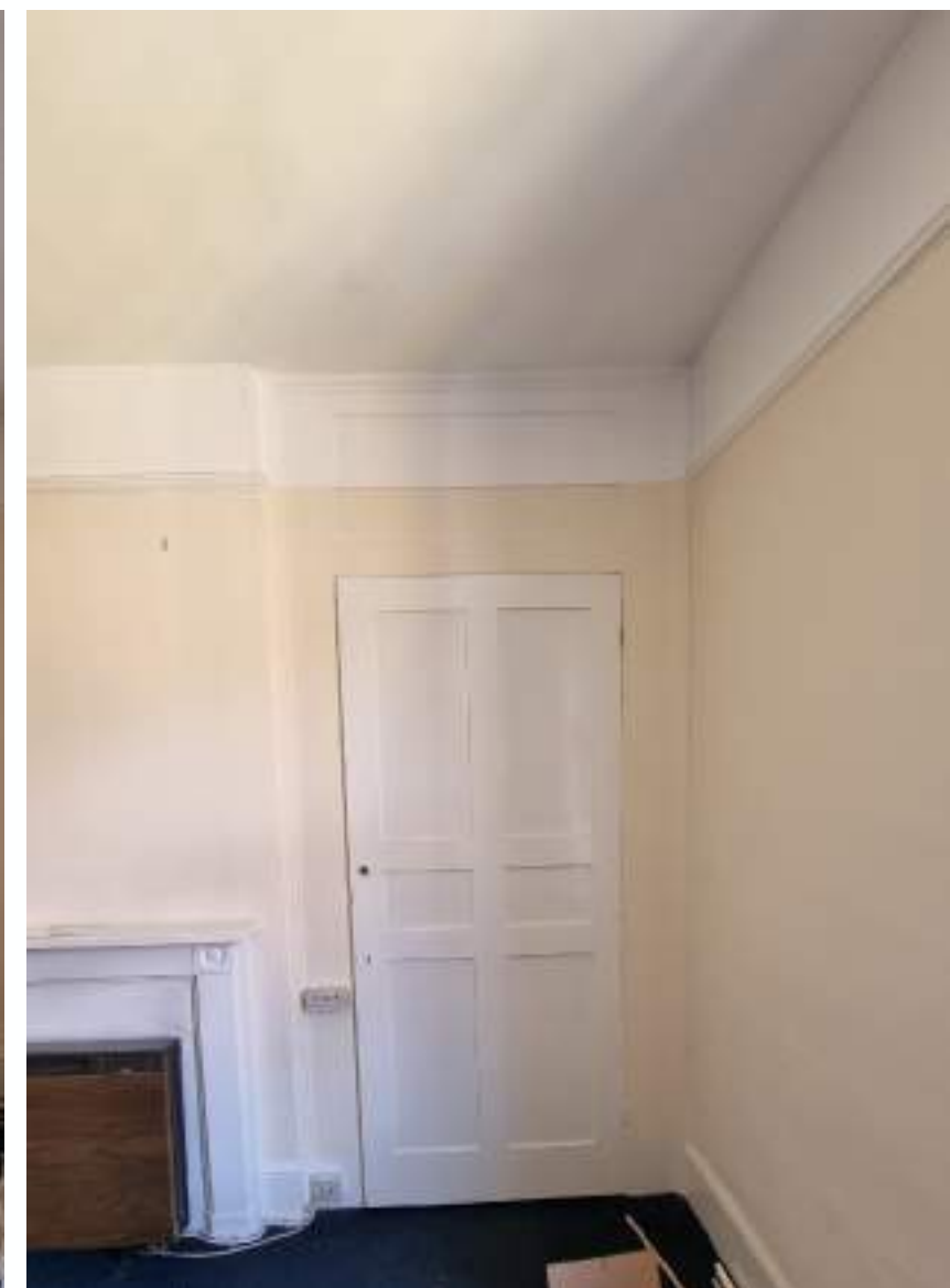
Existing door to store and chimney breast to be retained. Modern electric heater to be removed.
