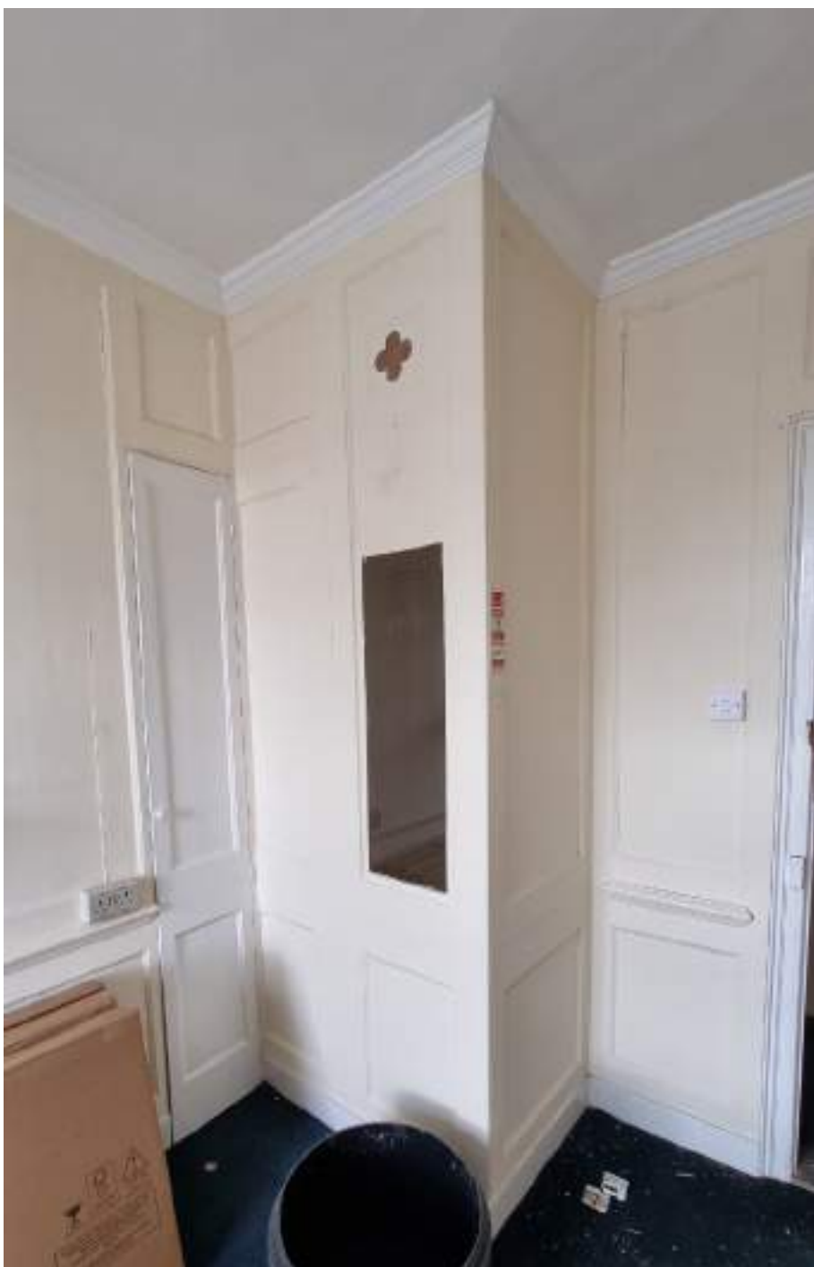
Thin timber panel wall to staircase, including small glazed panel.
