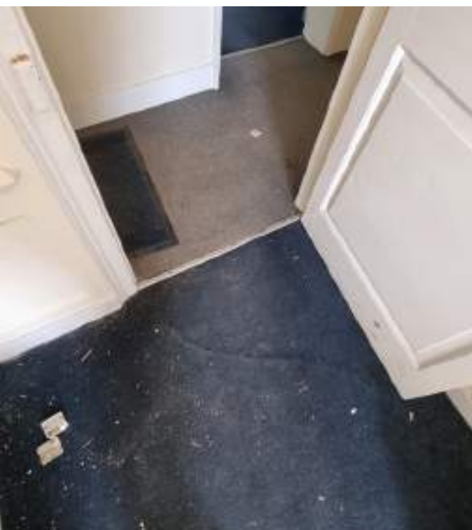
Existing carpet flooring replaced with carpet flooring.
