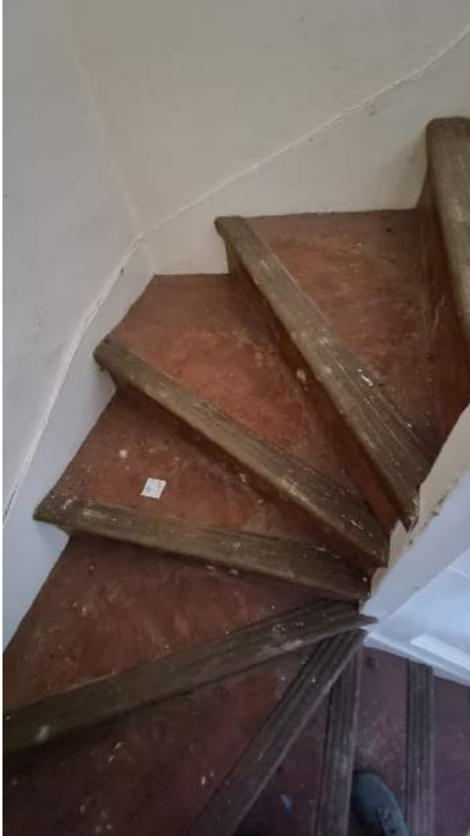
Stairs have modern finishes and skirting. New carpet finish proposed.
