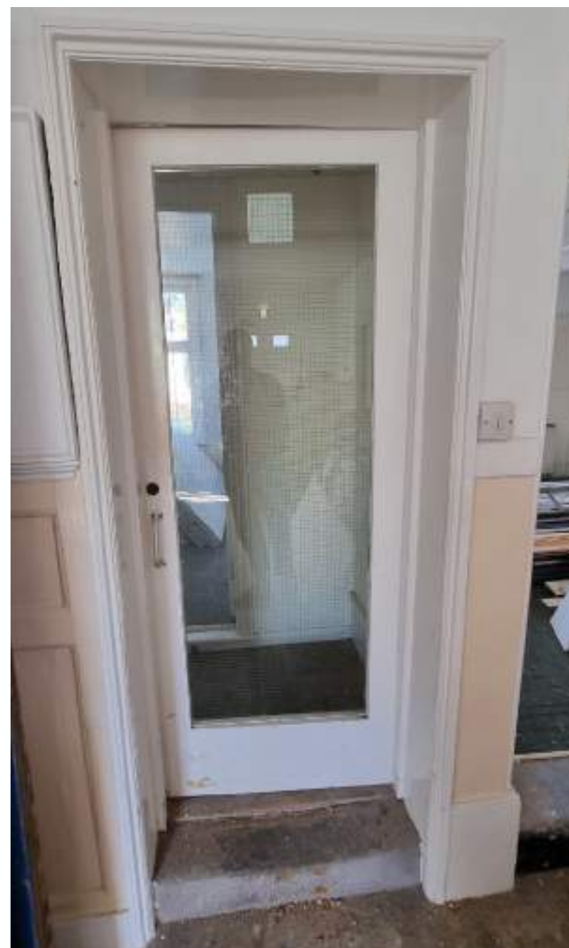
Door to flat 2 / existing corridor removed and closed off as per approved application.
