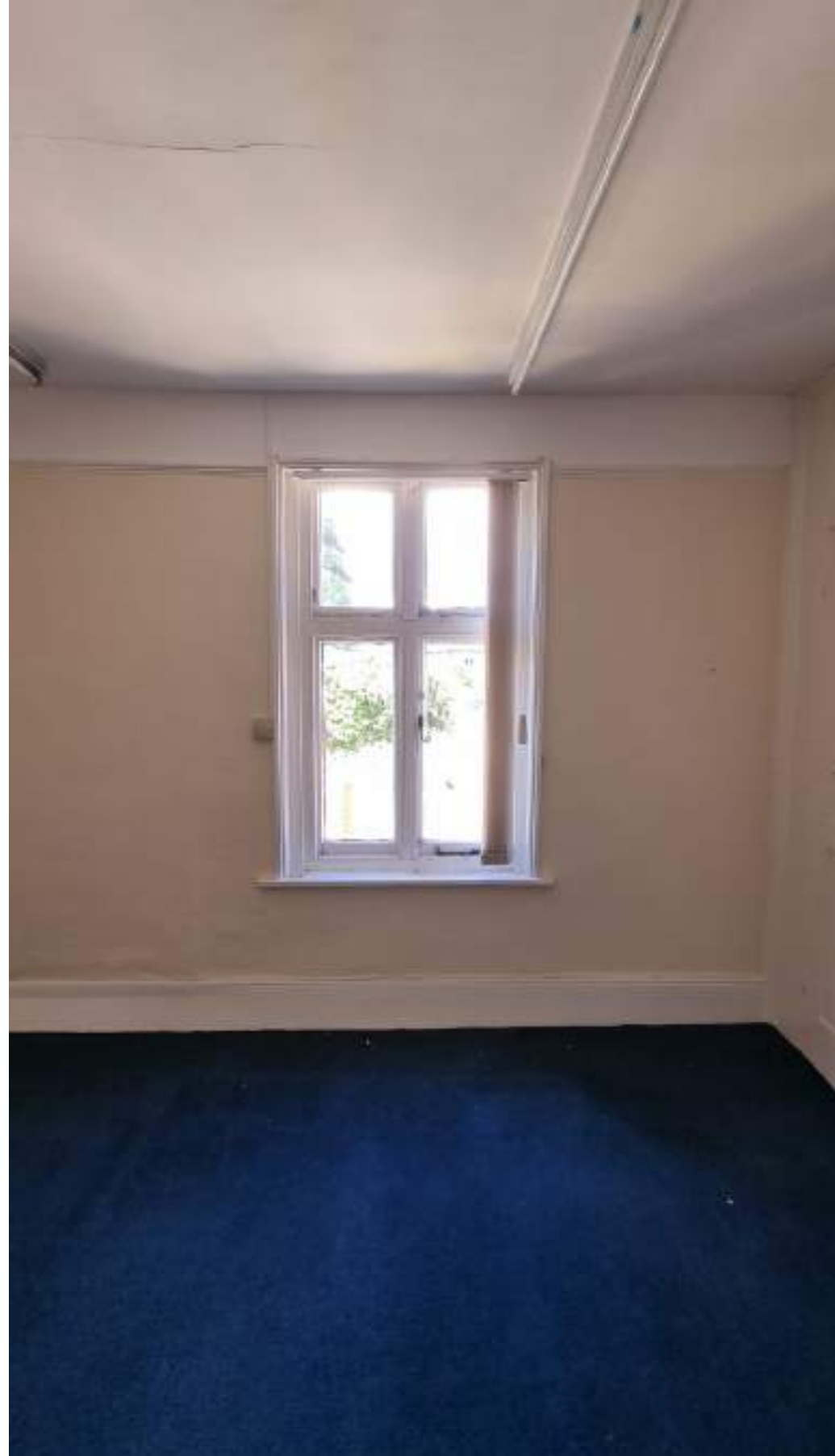
Existing ceiling and window
