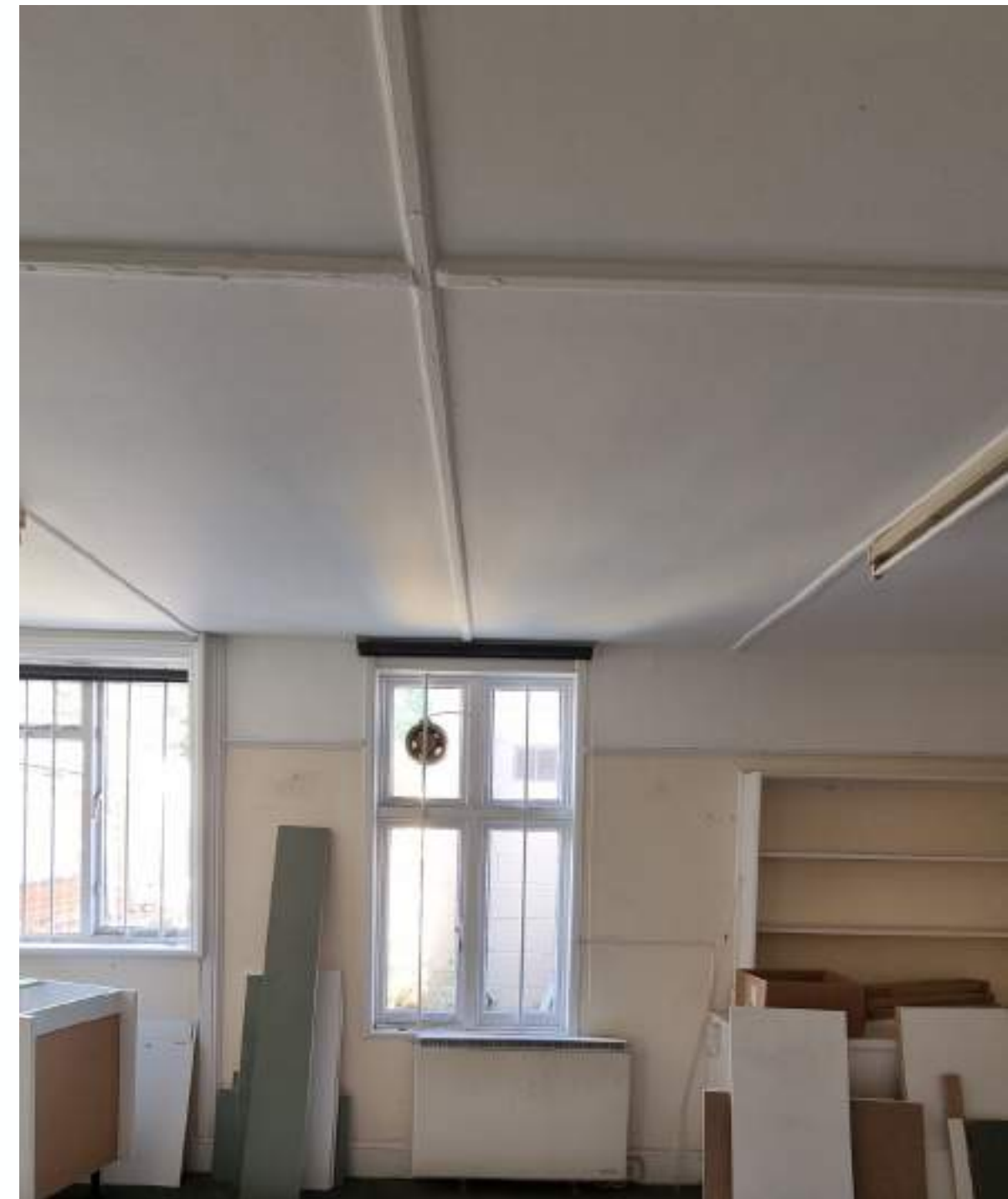
Minimal original features present. Timber detail to ceiling looks modern and of poor quality. Modern timber cabinet and electric heaters to be removed. Tall window removed as per approved application.
