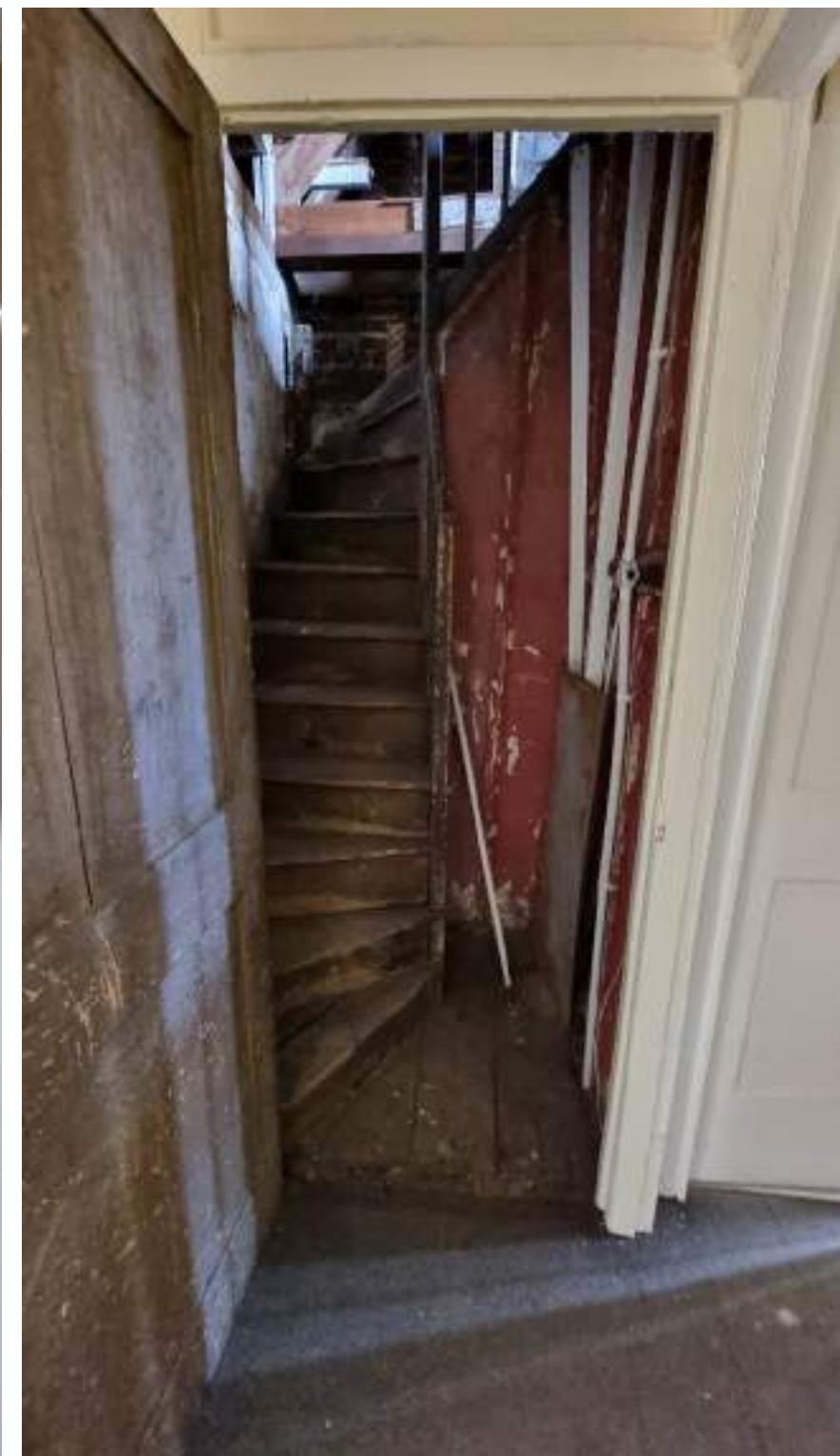
Stairs to loft storage
