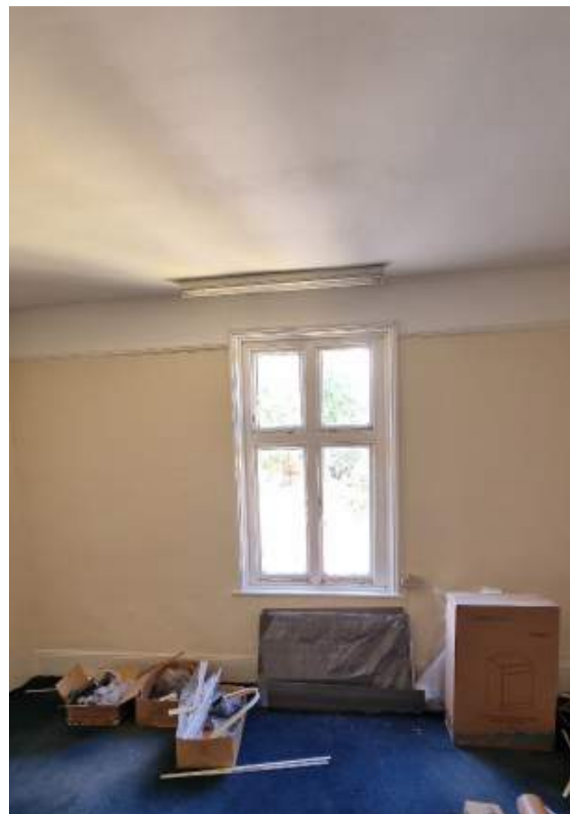
Existing ceiling and window to be retained.
