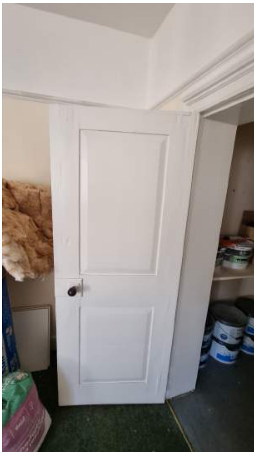
Door to store to be retained.
