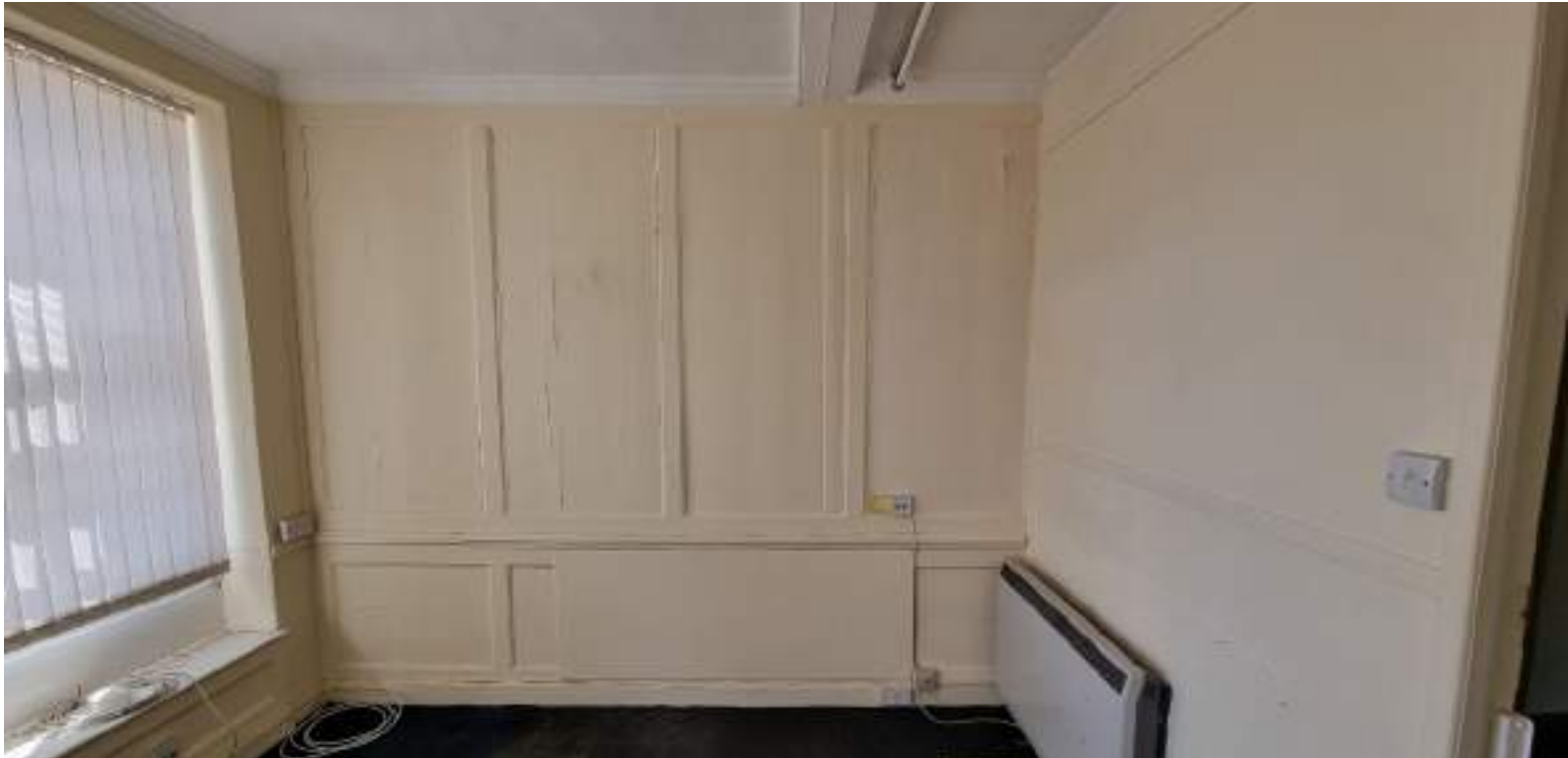
Existing timber panelling to be preserved. Modern electric heater to be removed.
