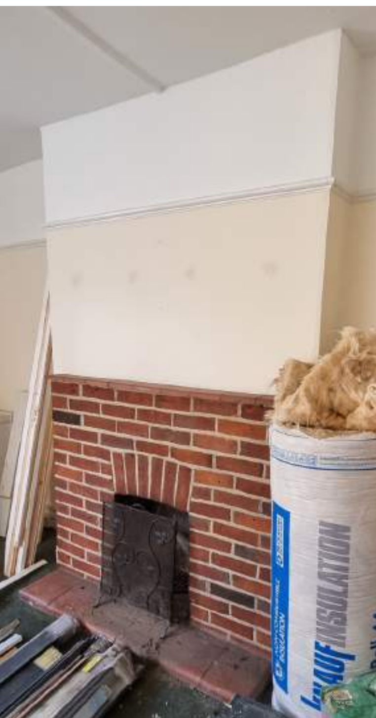
Chimney to be retained
