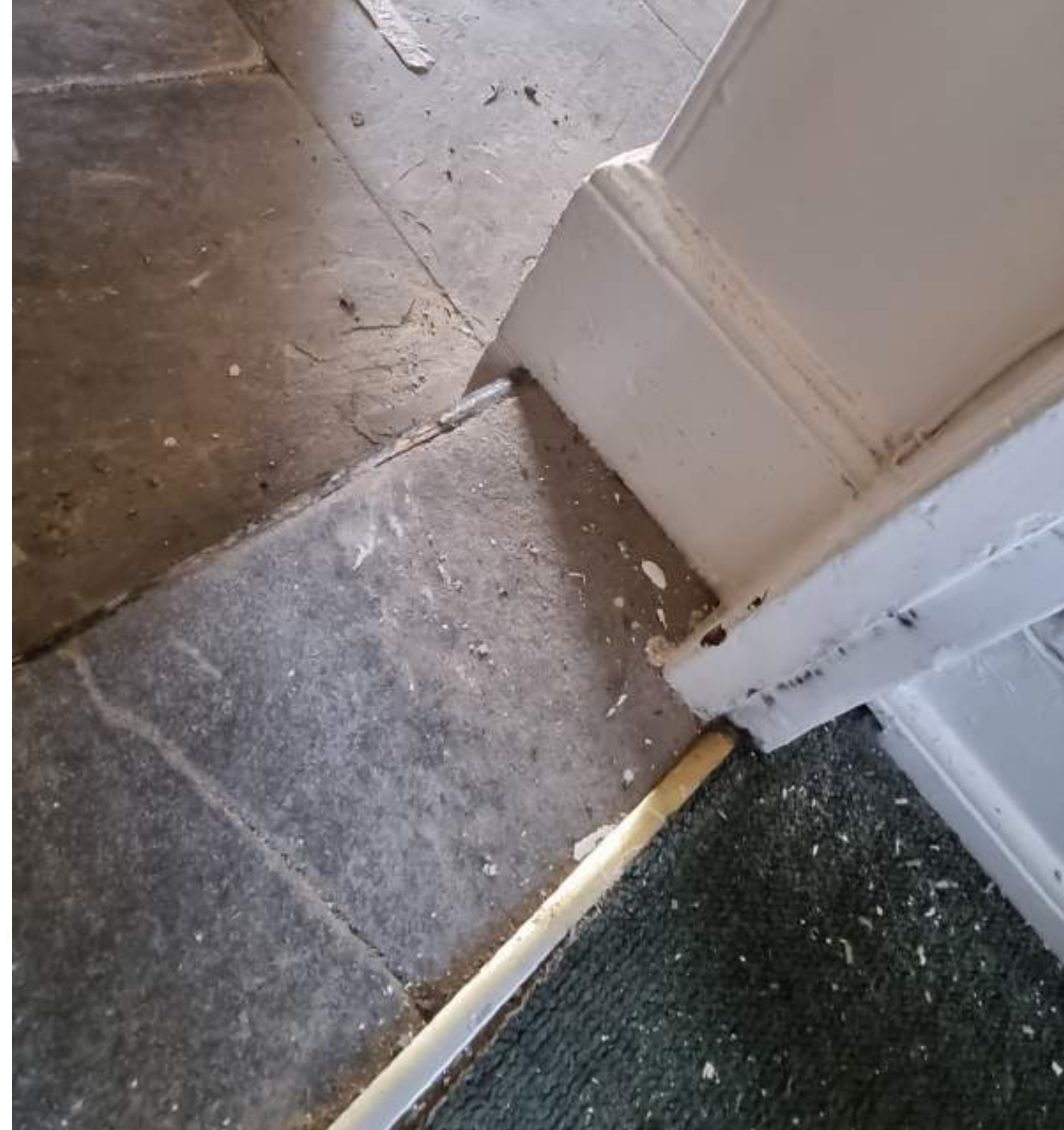
Existing stone pavers to ground floor office 2 (proposed living room to flat 2).
