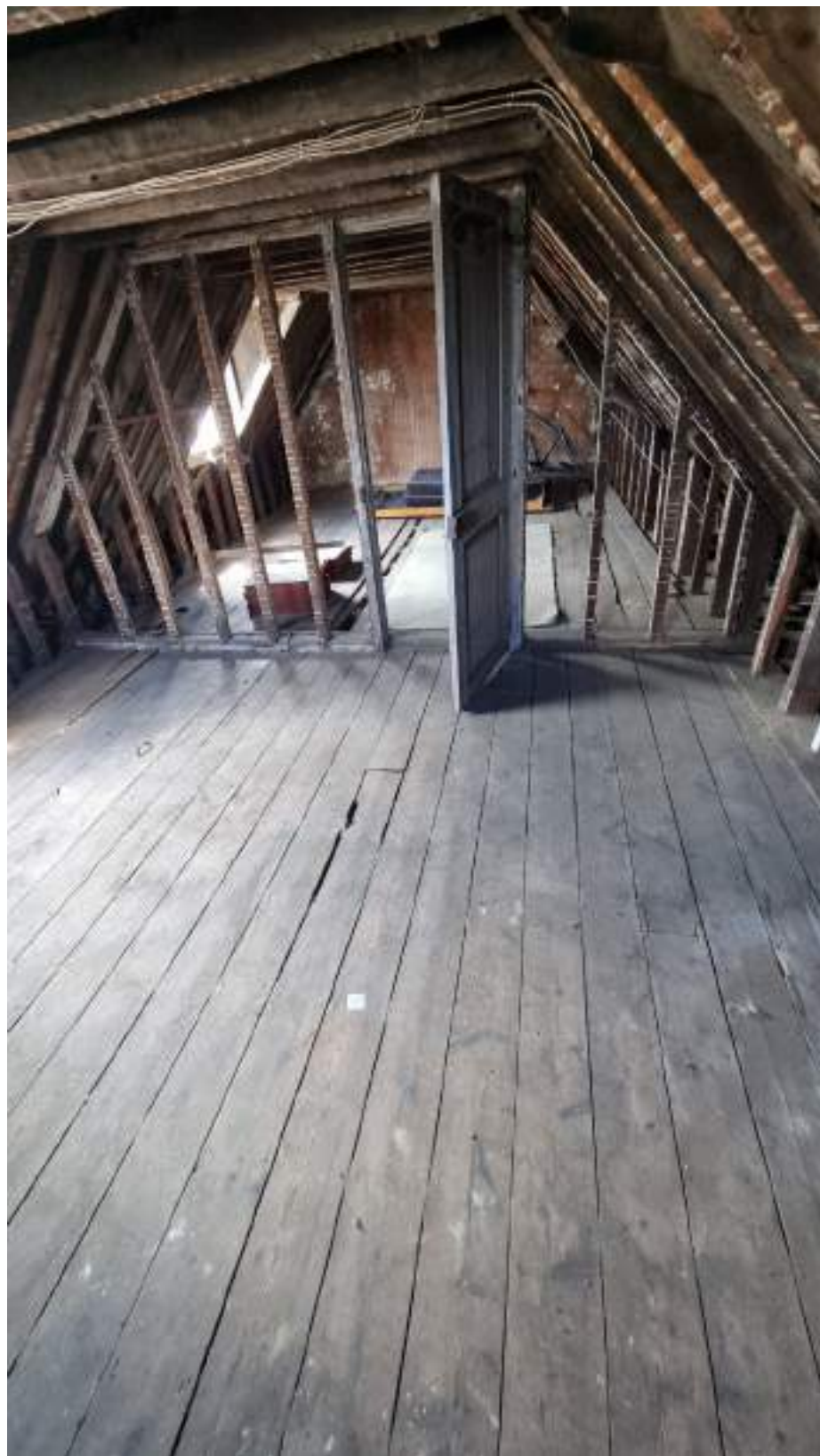
Unheated loft used as storage
