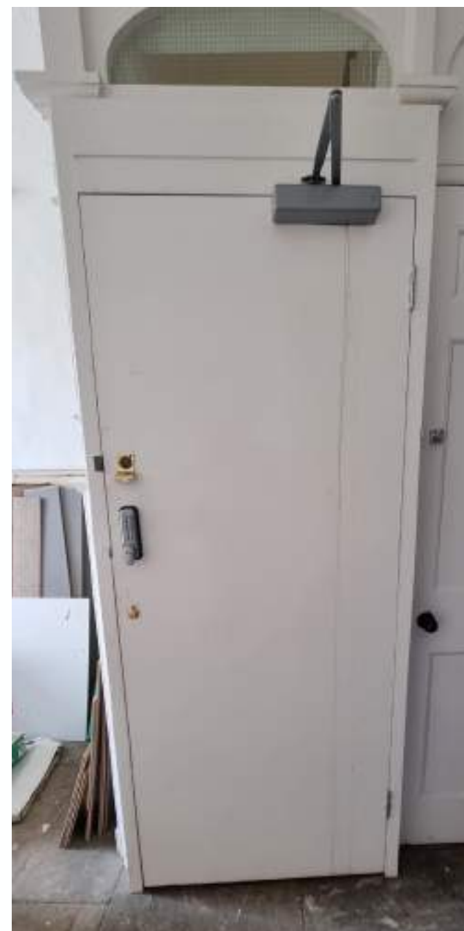
Modern door to entrance lobby to be removed as per approved application. Traditional timber panelling to staircase to be preserved.
