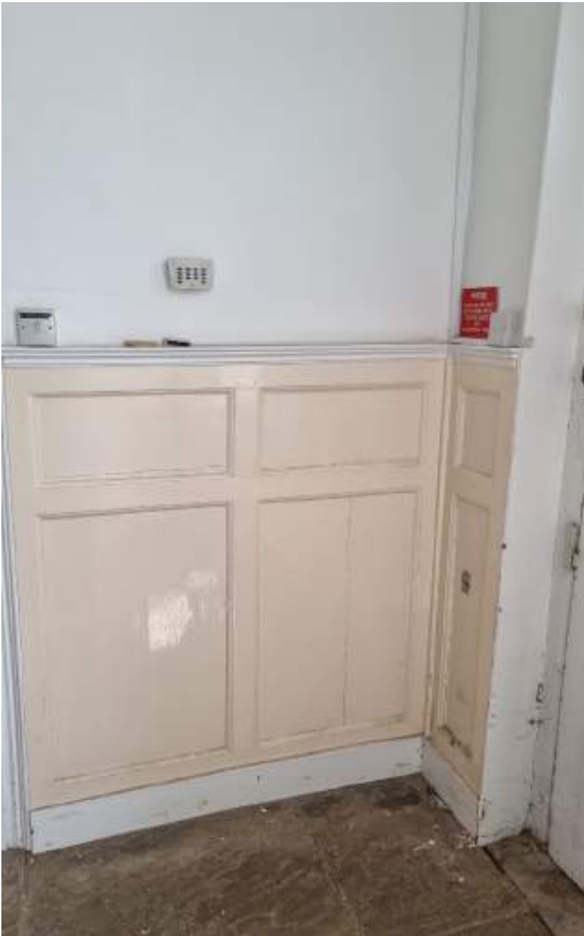
Existing timber panelling to be preserved
