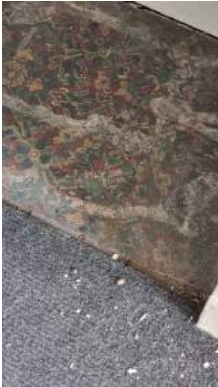
Existing timber floor under modern finishes.
