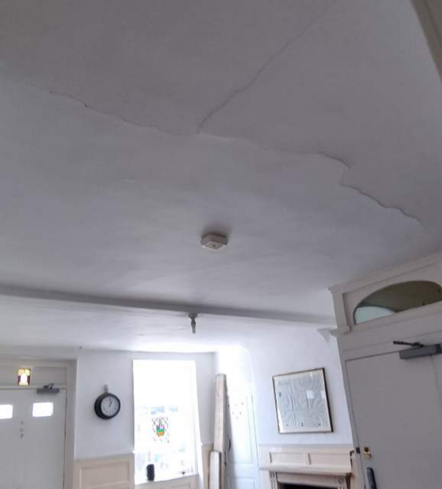
Lath and plaster ceiling to the entrance hall.
