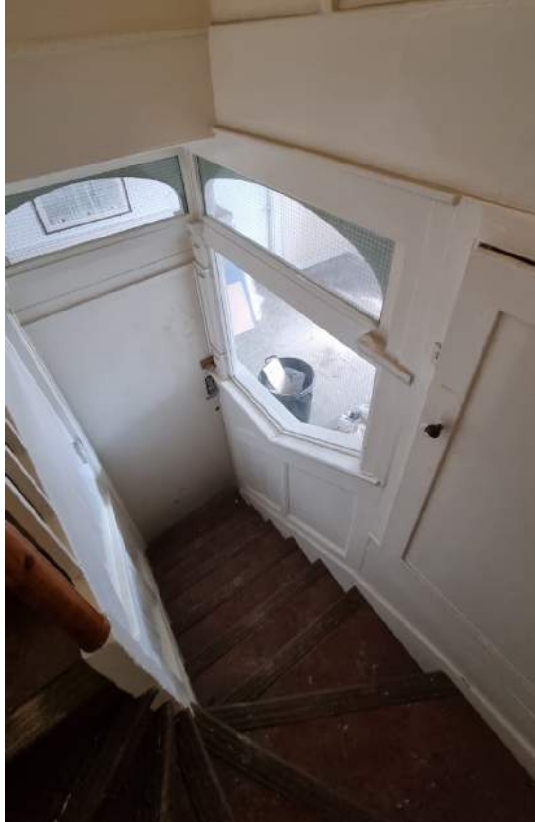
Modern door to the base of the stairs to be removed as per approved application.
