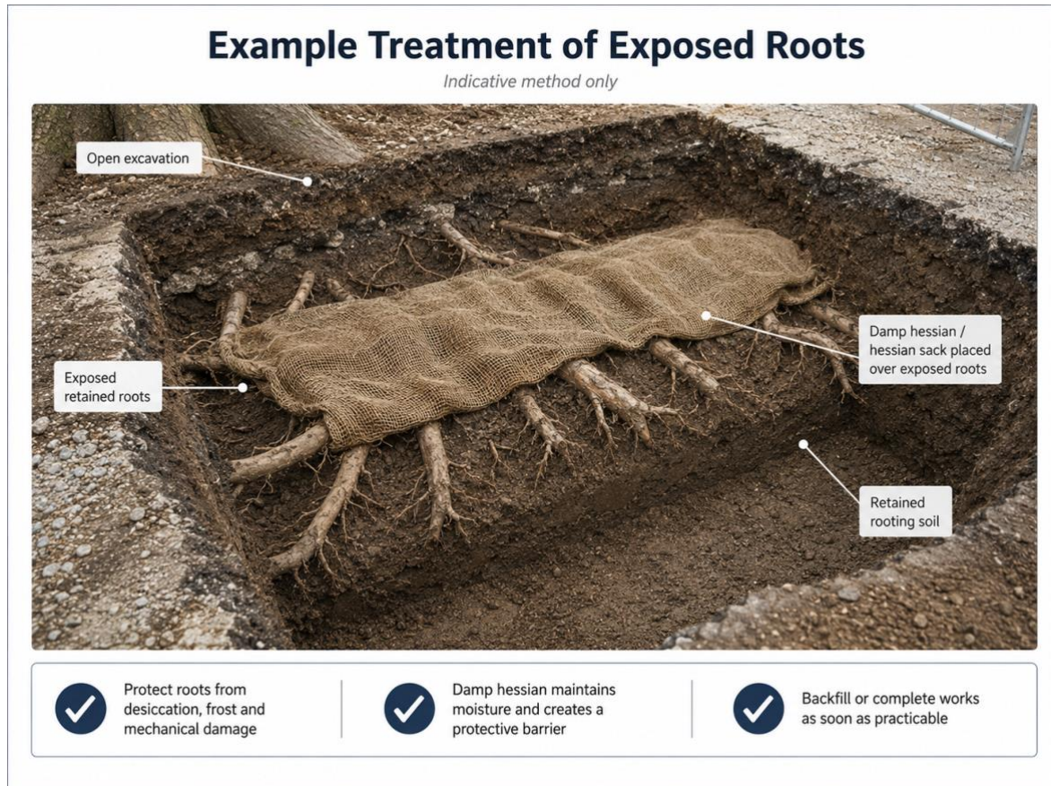
Figure 8– Example treatment of exposed roots within an open excavation. Retained roots are protected using damp hessian or similar breathable material to reduce desiccation, frost exposure and mechanical damage.
