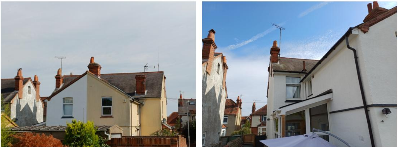
Figure 3 - Existing Roof Site Photos (4 August 2026)
