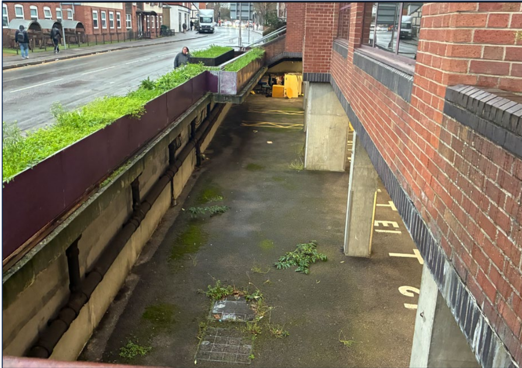
Figure 2-3 Undercroft Parking (Crown Street on the left of the image)
