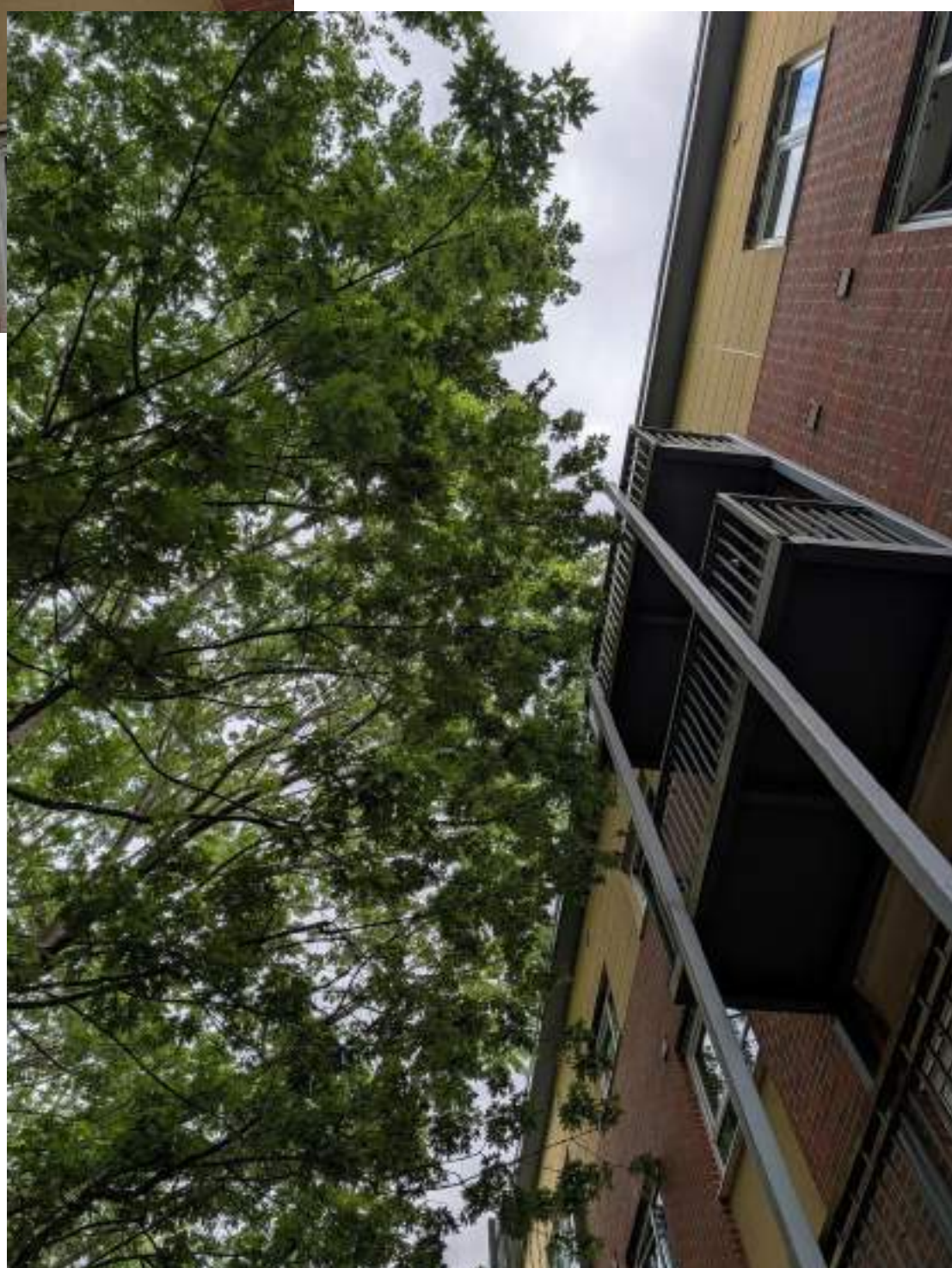
B.8/9 – T004/5 Showing proximity of limbs to building and balconies.
