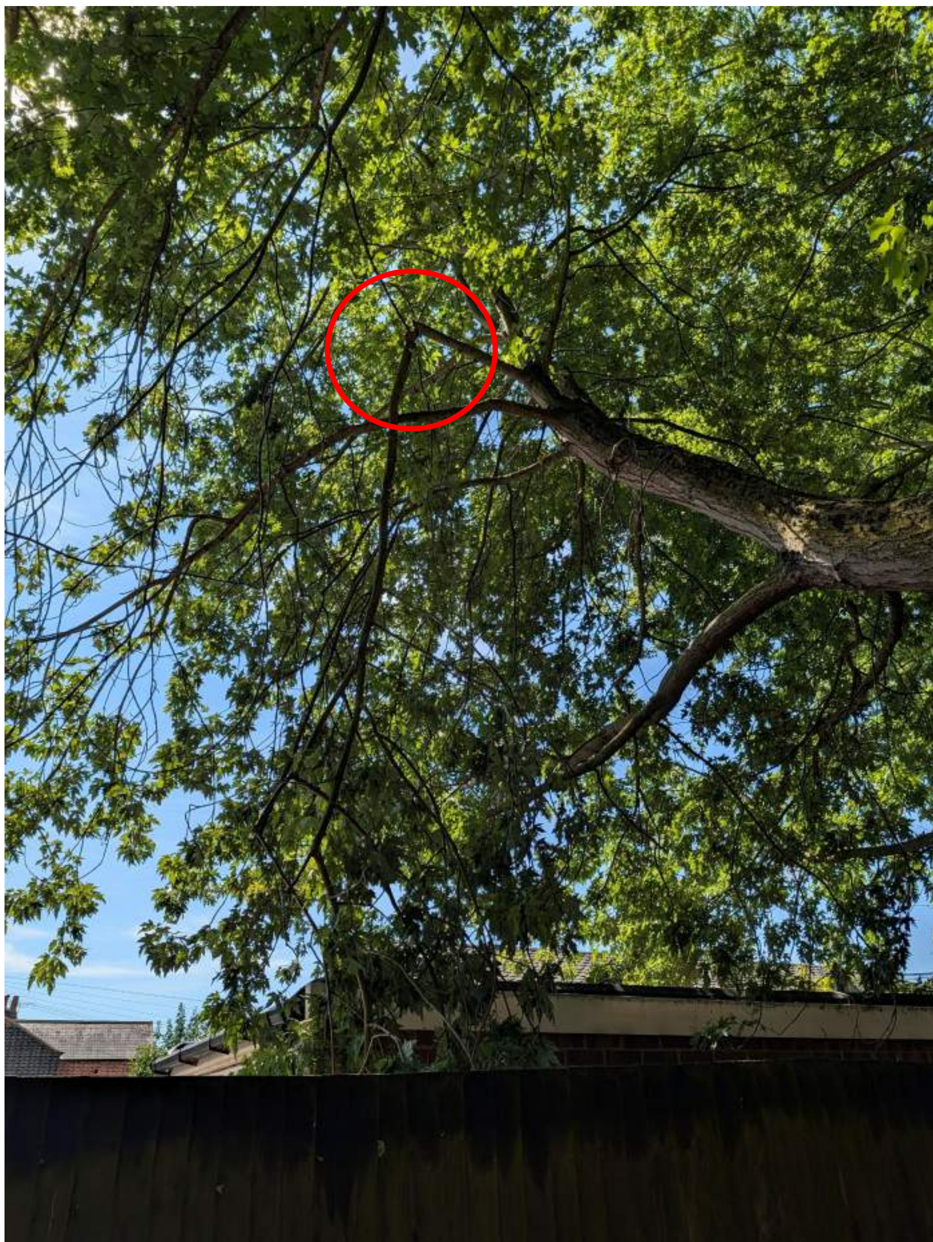
B.21 – T012 showing multiple limbs interfering with building and highlighted snapped hanging branch.
