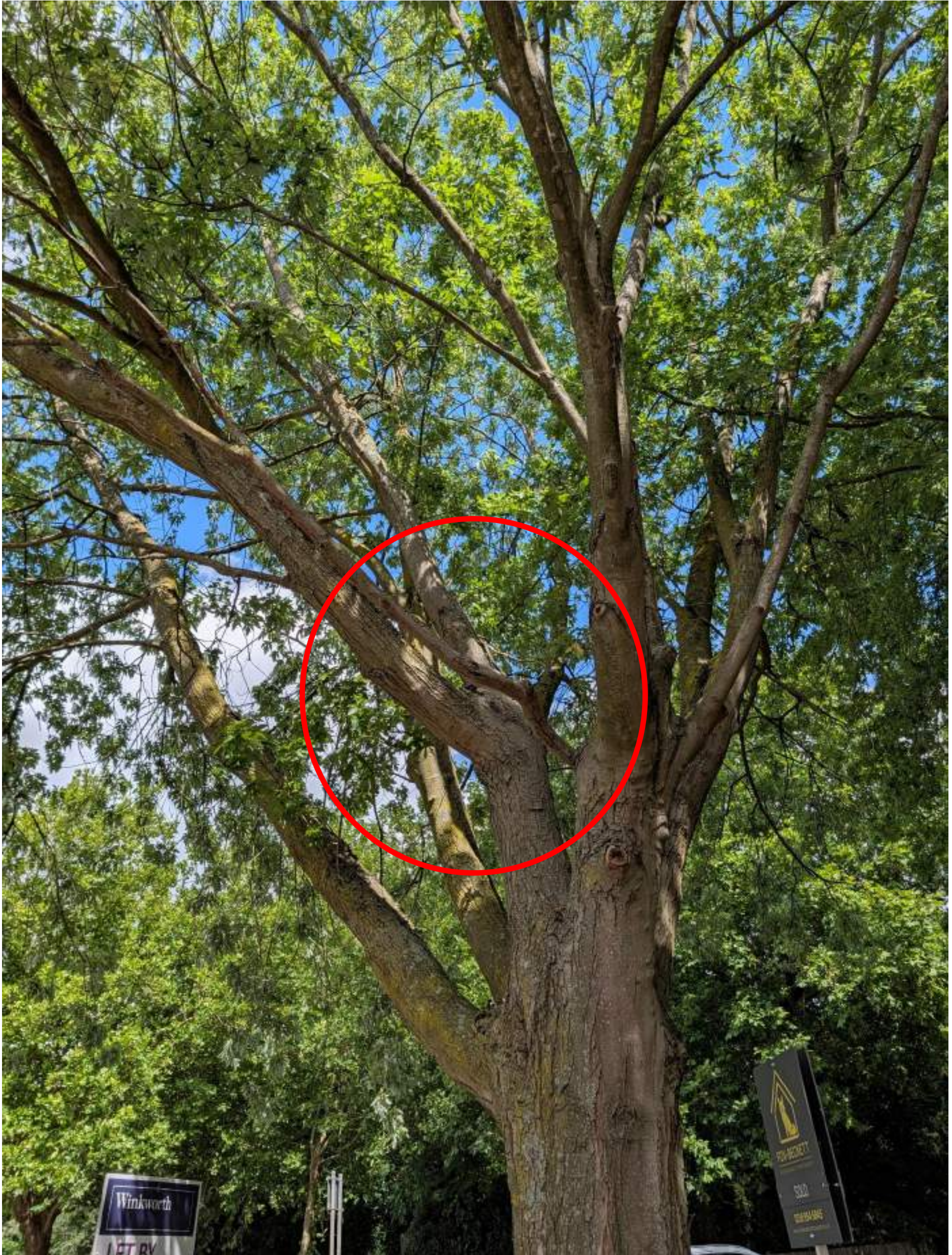
B.1 – T001 image highlighting significant deadwood over parking bay.
