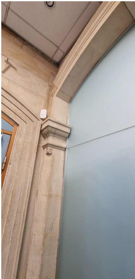
Figure 4: Photos showing the existing stonework alterations to embed the glazing frame where the stone details protrude from the face of the column.
