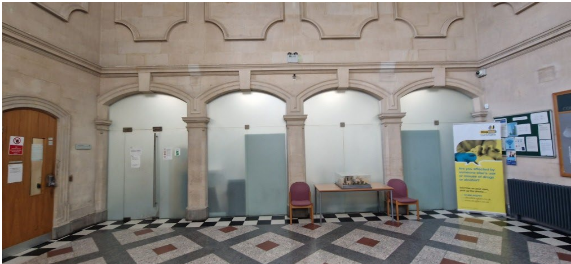
Figure 1: Photo showing the east elevation of the Entrance Foyer.
