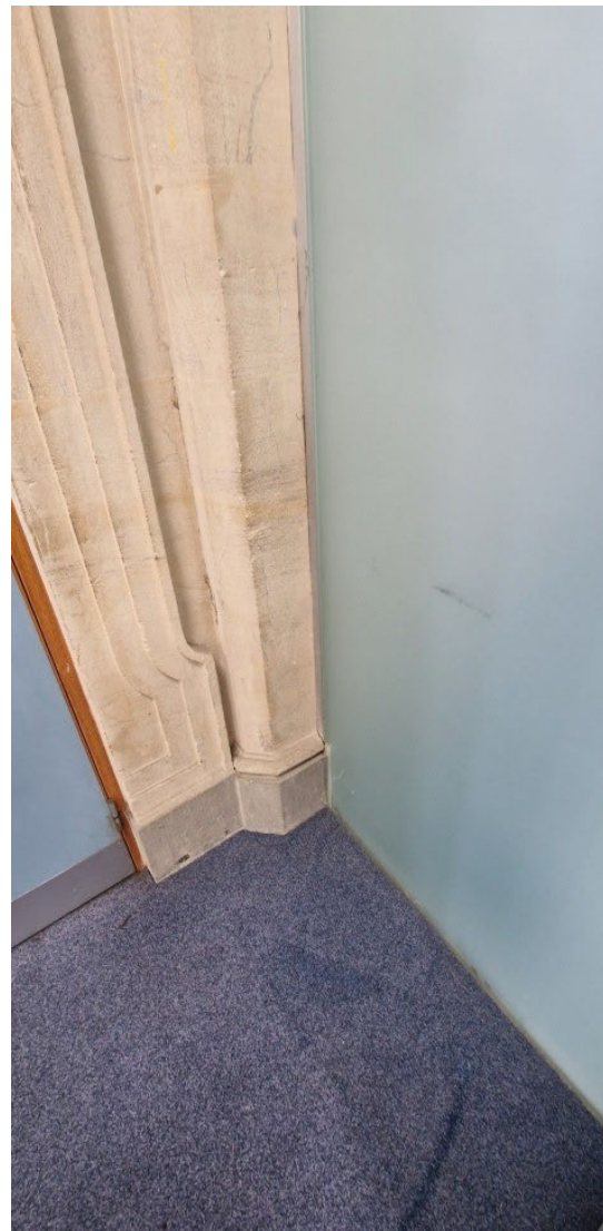
Figure 4: Photos showing the existing stonework alterations to embed the glazing frame where the stone details protrude from the face of the column.
