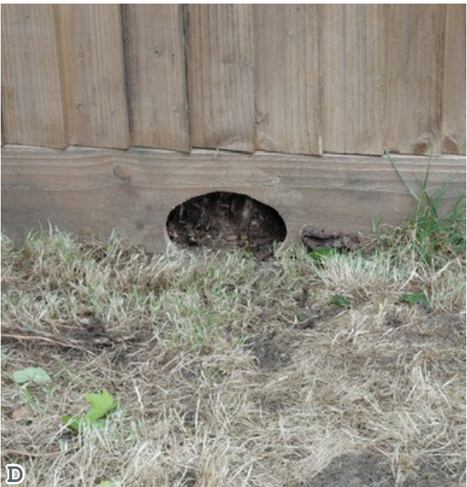
D Mammal Gap - Opening in fence at ground level to allow wildlife such as hedgehogs to pass through
