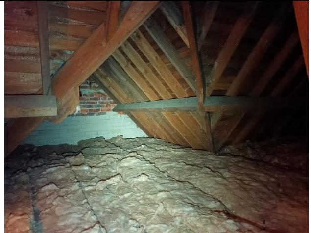
PHOTOGRAPH 12– ROOF VOID EXTENDING INTO PITCHED ROOFED AREAS
