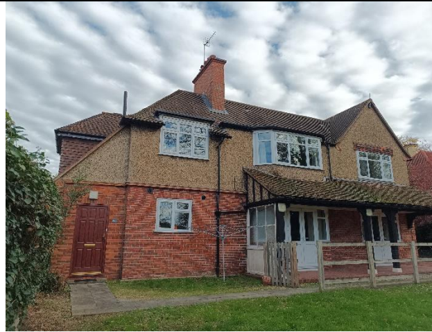
PHOTOGRAPH 7– SOUTH-WEST ELEVATION OF THE PROPERTY WITH SMALL AREA OF TILE HANGING ABOVE A WINDOW
