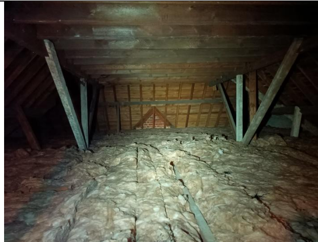
PHOTOGRAPH 11– CENTRAL FLAT ROOFED SECTION OF THE ROOF VOID
