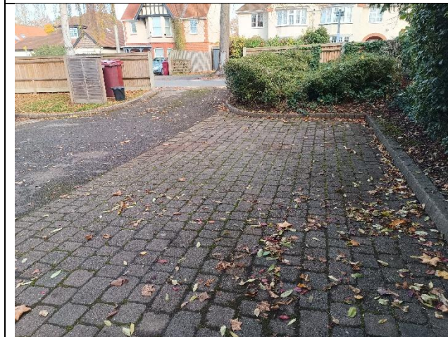
PHOTOGRAPH 3– DEVELOPED LAND; SEALED SURFACE AND ADJACENT INTRODUCED SHRUB IN SOUTH-EAST OF THE SITE
