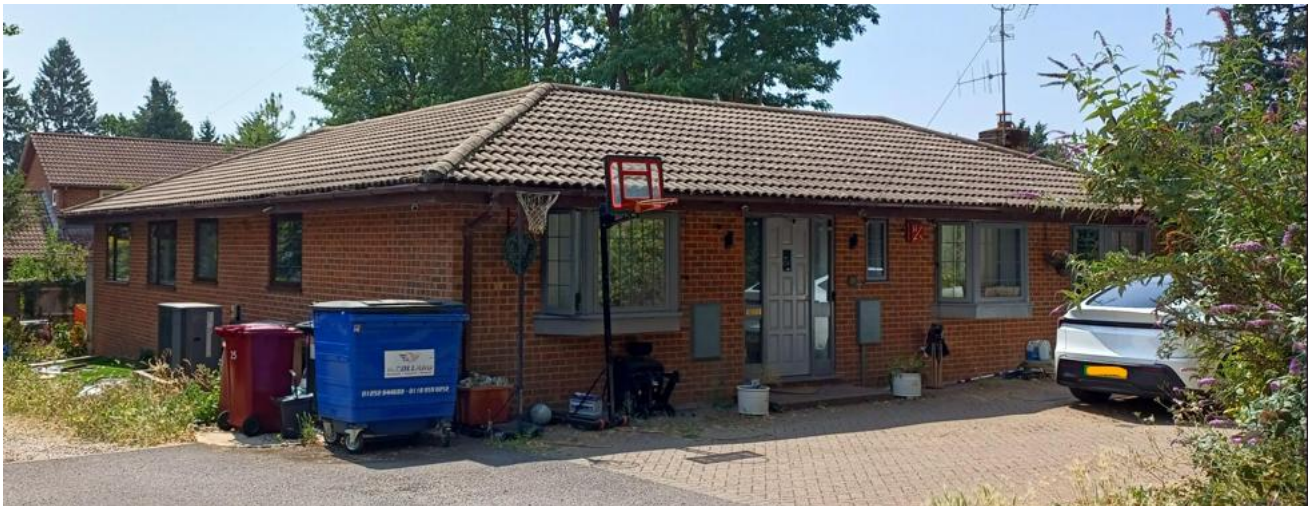
View of 22 Queensborough Drive, taken by the case officer on 10 th July 2026
