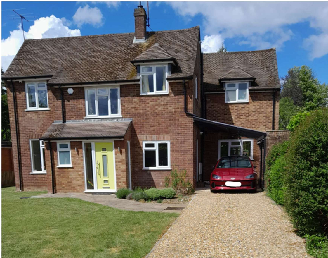
Looking towards front elevation
