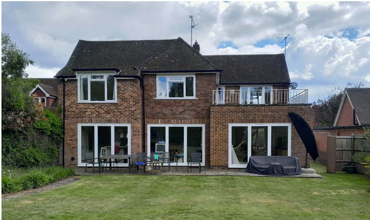
Looking towards existing rear elevation
