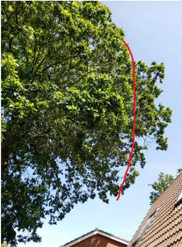
Figure 6 (Oak T1 of Report; T2 of TPO): reduce branches growing towards No. 23 to provide clearance of the roof
