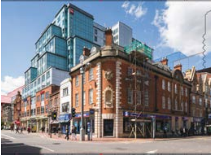
Figure 7.7 Emerging context as part of Station Hill Phase 3, seen from Queen Victoria Street and Station Road junction [taken from ES and TVIA submitted as part of the application]
