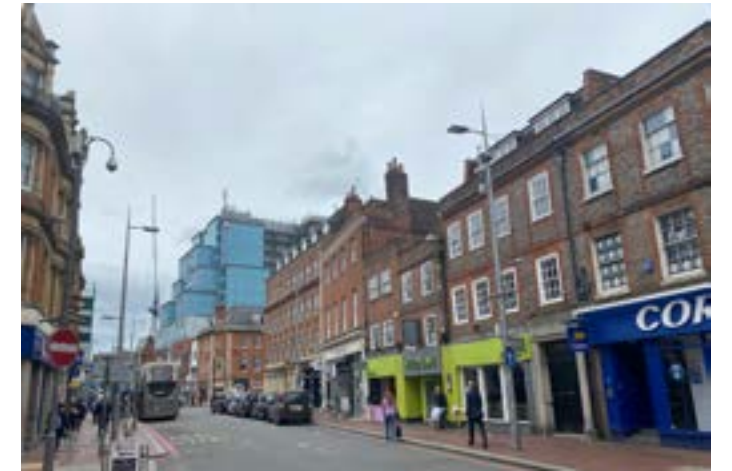
Figure 4.3 Site overlooking new development at Former New Cross Hospital).
