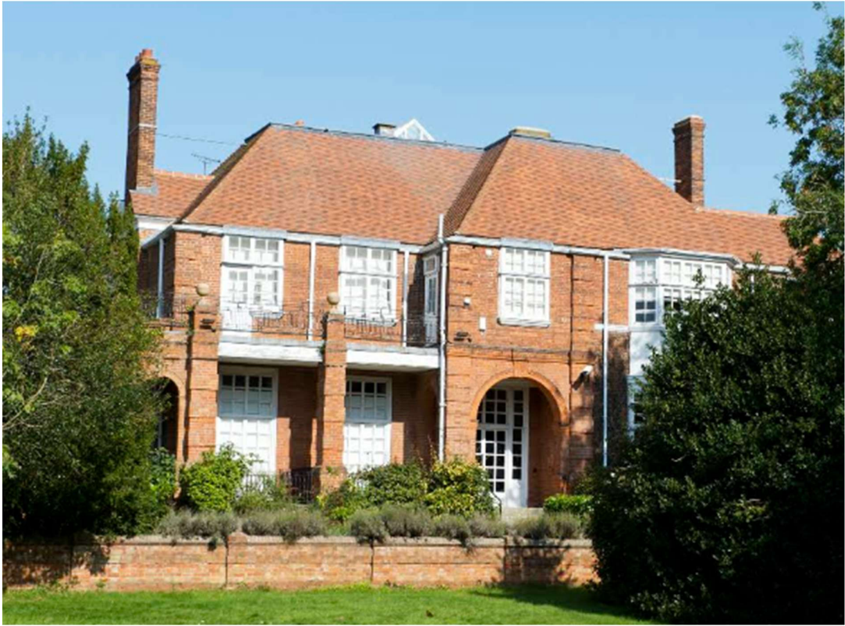
Rear elevation of the Grade II Manor House (Highdown School)
