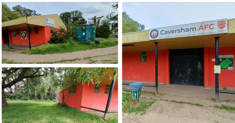
Figure 2 - Site visit photographs of building as existing
