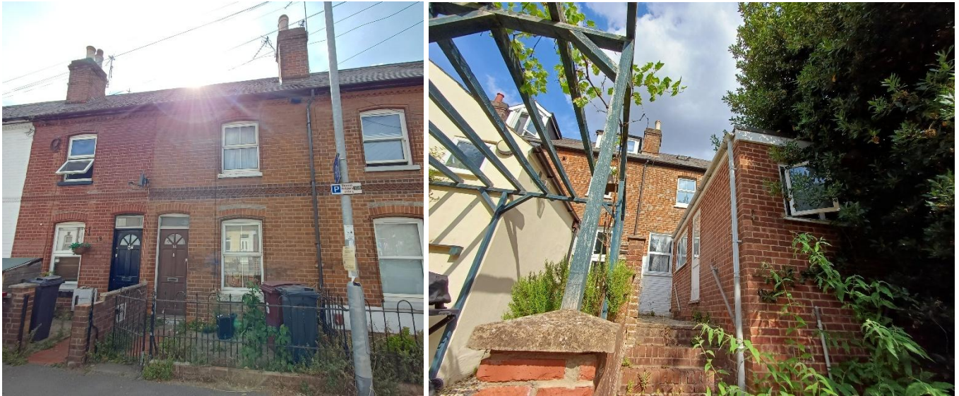
Front and rear views of 18 Elgar Road, taken on 07/24/2026
