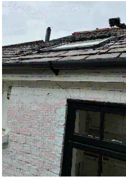
Rooflight internal & external Views
