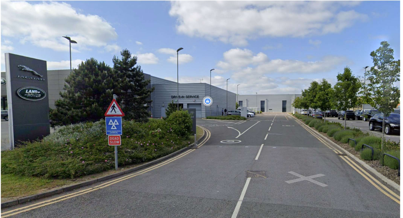
Looking due north towards drive-in-service and workshops from entrance off Bennet Road
